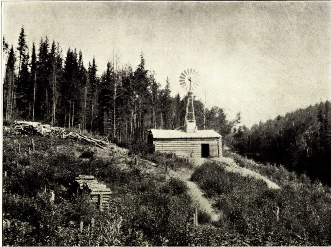
Shaft House, Height of Land Mining Company.
