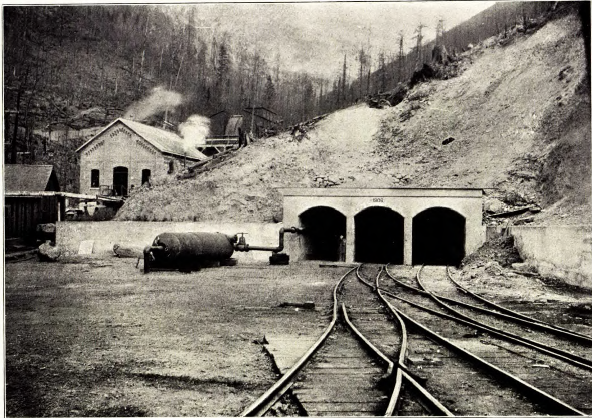
Hosmer mines: main tunnel, Hosmer, B.C.
