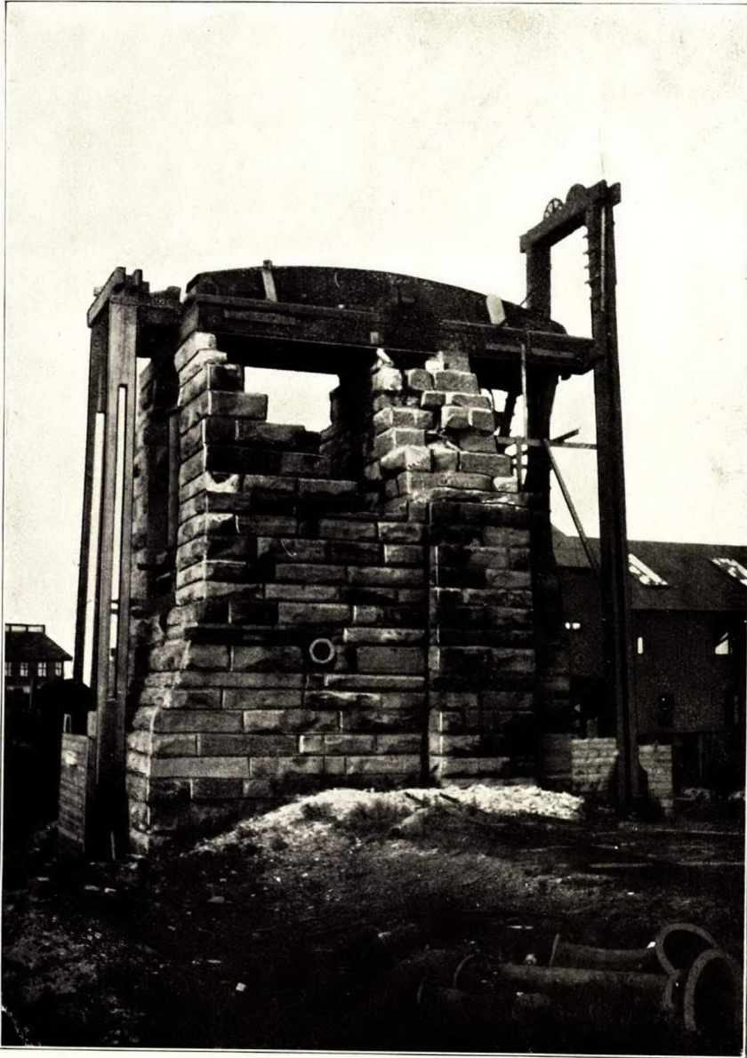
Old Cornish pump, Foord colliery, Stellarton, N.S.
