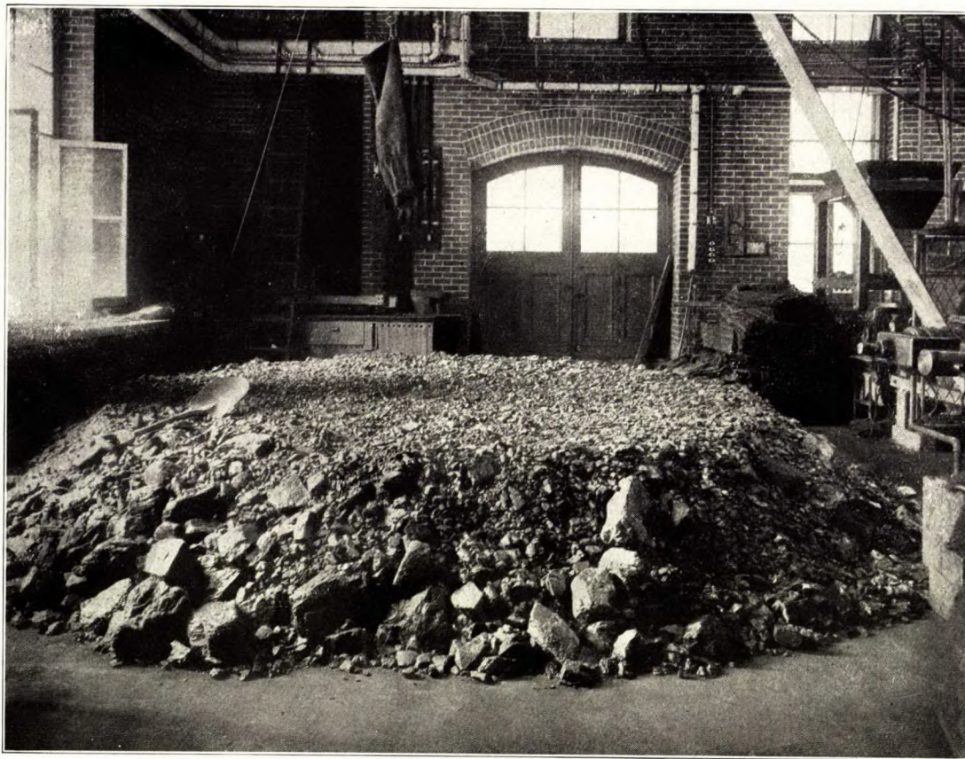
Sampling. A flattened cone of coal. Department of Mining and Ore Dressing, McGill University.
