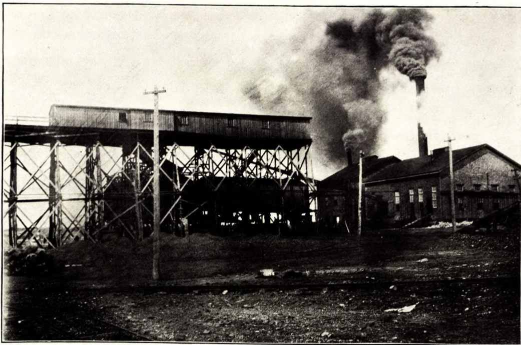
Tipple and Power House. Port Hood Coal Co., Inverness county, N.S.
