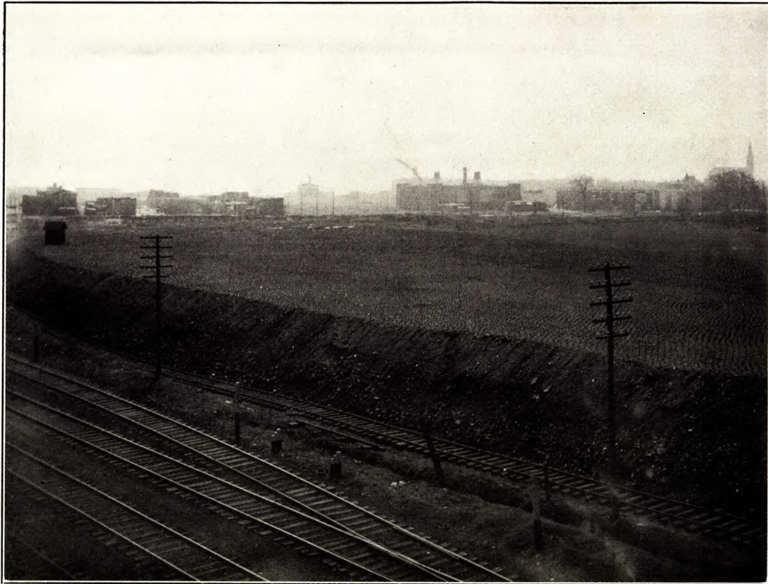
Ventilated coal pile at Montreal. General view.
