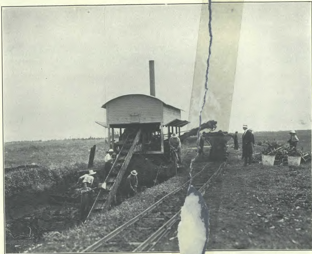
30 ton "Anrep" Peat Machine : end elevation, showing El Trenching Operations, and Track.
