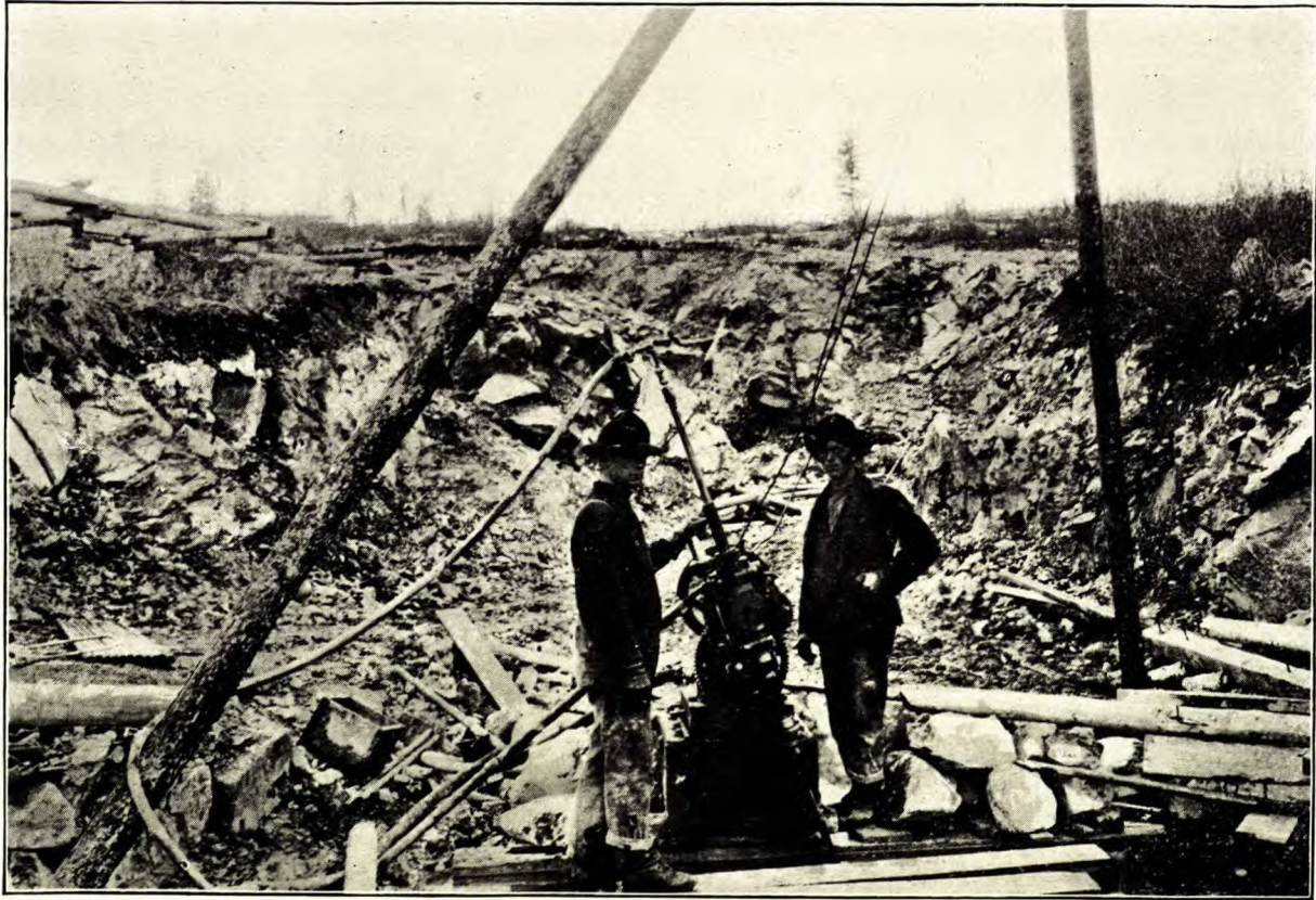
Diamond Drilling at the Montreal Mine.
