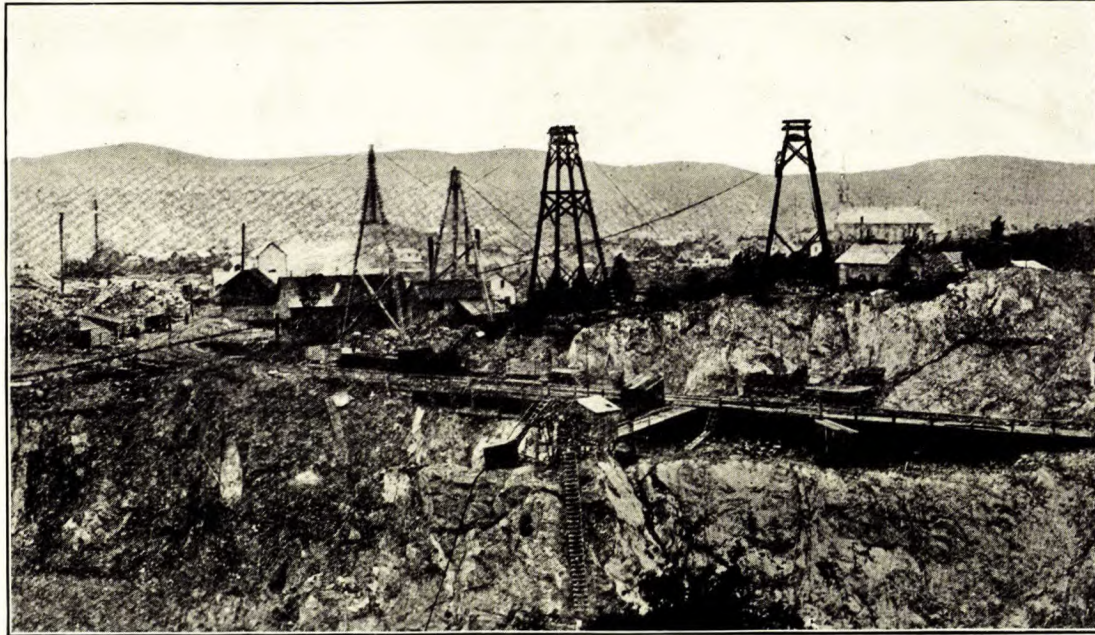
Arrangement of Cable Derricks and Tracks near Border of Pit. King Bros.' Mine, Thetford.
