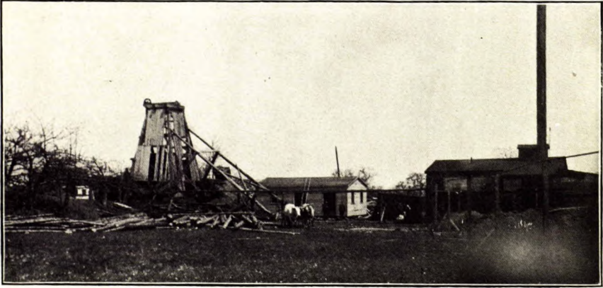
(a) Wheelock shaft house: Torbrook district.
