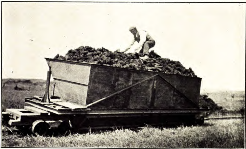
Car for transport of Dried Peat, Aamosen, Denmark.
