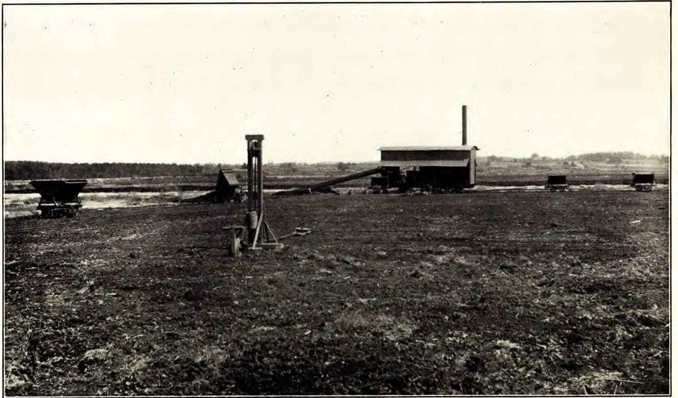
Cable Transportation of Machined Peat at St. Olof, Sweden.
