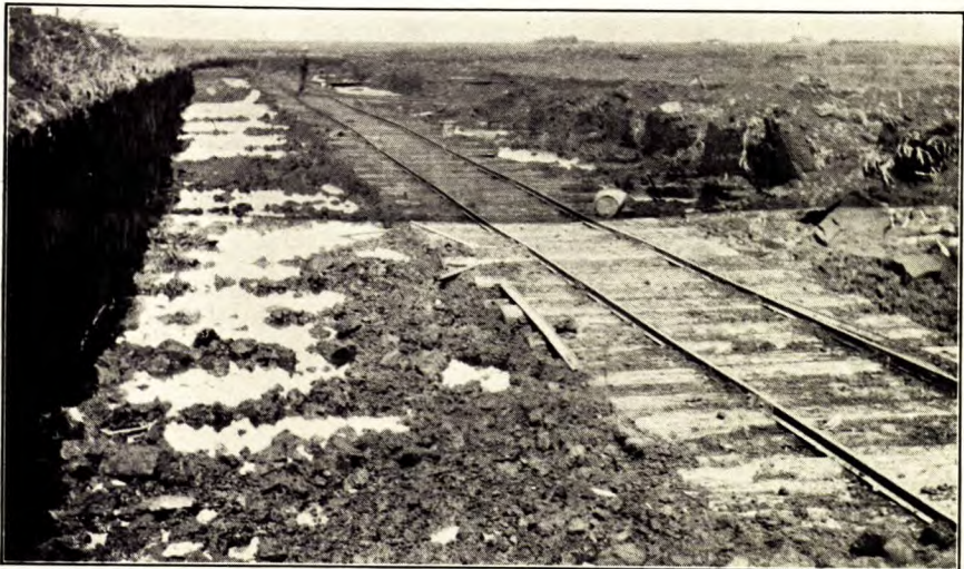
Working Trench at Ökaer, Denmark.
