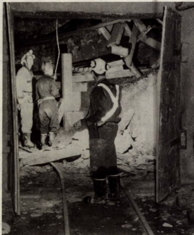
Both MRL's Elliot Lake Laboratory and MRL's Rock Mechanics Laboratory are investigating the causes of rockbursts in underground mines
