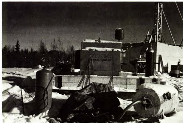
Field-testing standard and experimental oil-fired water line heaters
