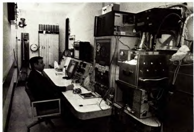
Diesel control room at CEAL
