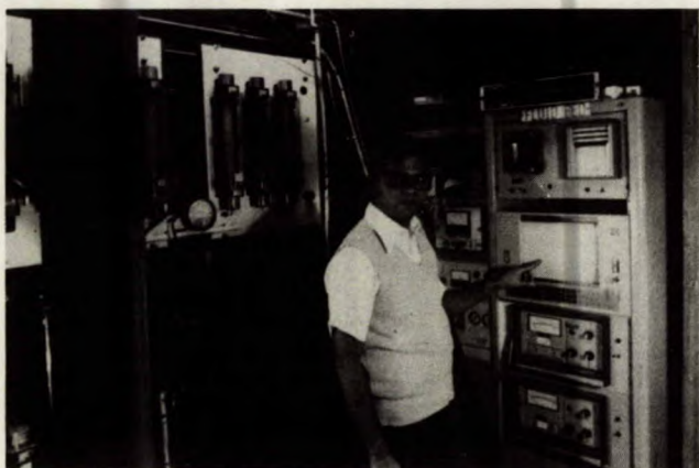
D. Desai, engineer, examines data from fluidized-bed combustion tests using Canadian coal
