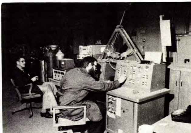
Researcher G. Lobay (R) and technologist S. Ferguson operate control console of explosive atmospheres tests facility
