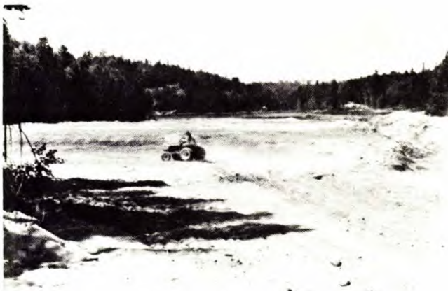
Preparation of tailings for revegetation
