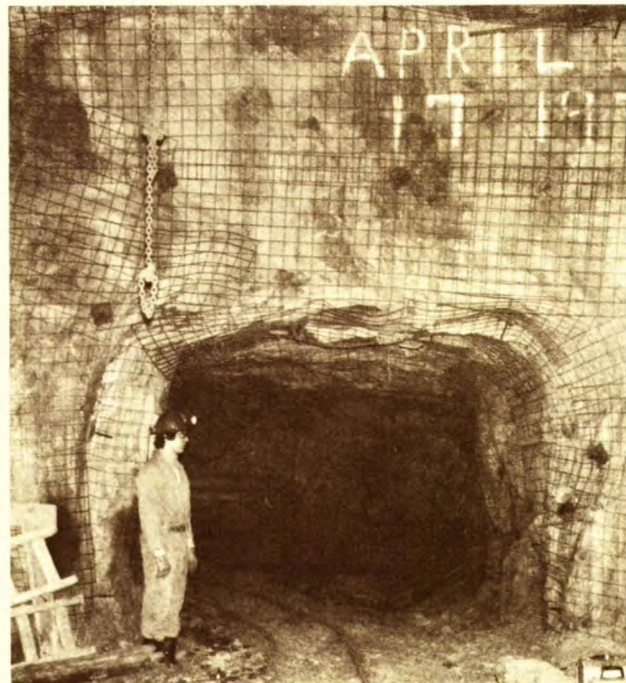
Fig. 19 - Section of test chamber being investigated for underground storage of nuclear waste
