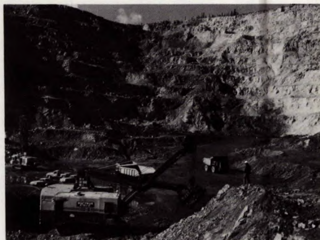
Figure 6 — CANMET's multi-million-dollar Pit Slope Project, initiated in 1972 in an effort to develop improved open pit mining procedures, is nearing completion with production of a ten-chapter engineering manual. Photo — George Hunter
