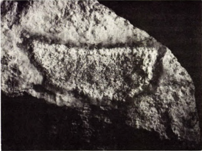
Fig. 3 - A fracture through 45-year old concrete, from a river pier, containing reactive calcitic Potsdam sandstone aggregate. Translucent siliceous gel (with desiccation cracks) migrated along the fracture from reacting aggregate. The porcellaneous deposit lying within the dark clarified rim contains much calcium, either derived from the calcite or transported. Mag 3x.
