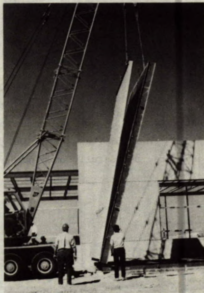
Fig. 11 - Erection of precast panels, Calgary, Alta.
