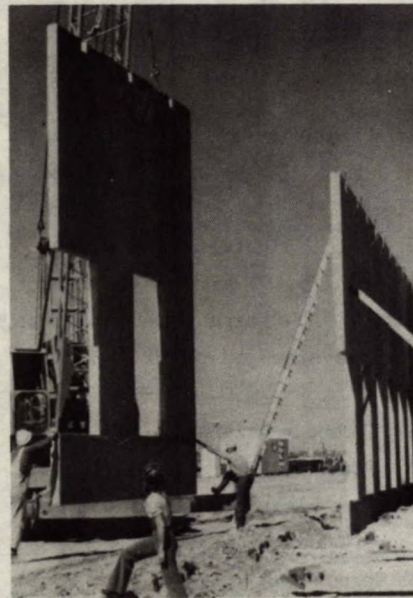
Fig. 11 - Erection of precast panels, Calgary, Alta.
