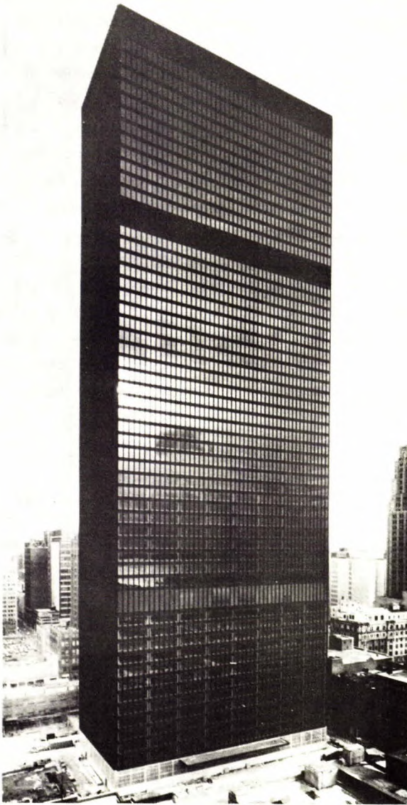
Fig. 14 - Toronto-Dominion Bank Centre, Toronto, Ontario
