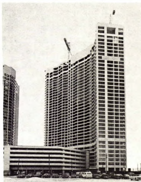
Fig. 9 - Harbour Square Apartment Complex, Toronto, Ont.
