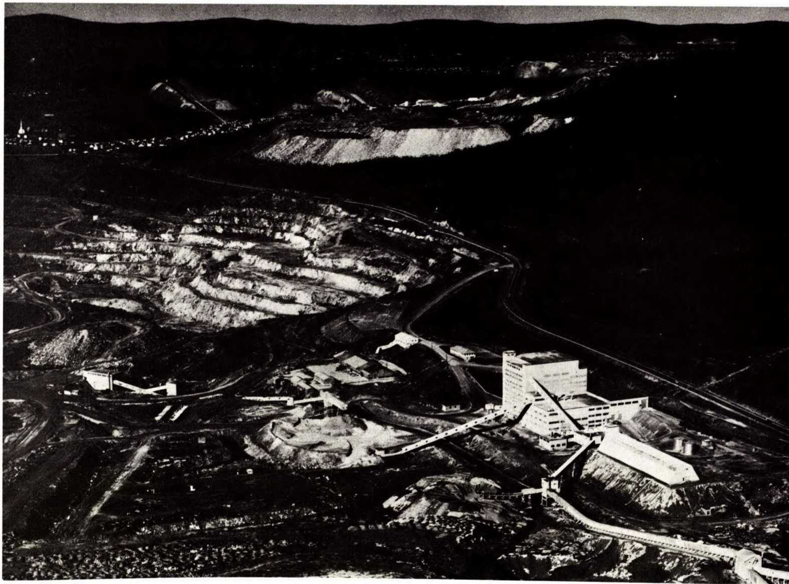
Figure 4. Open pit and mill of Lake Asbestos of Quebec Ltd. at Black Lake, showing waste rock dump and mill tailings (photo by George Hunter).
