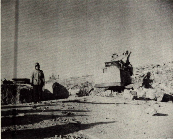
Fig. 14 - A 3-m upheaval and floor cracking in an open pit mine indicating the presence of high horizontal stresses (From "Pit slope manual, Ch 5 - Design" by D.F. Coates; CANMET Report 77-5 , EMR; 126 p; 1977.)
