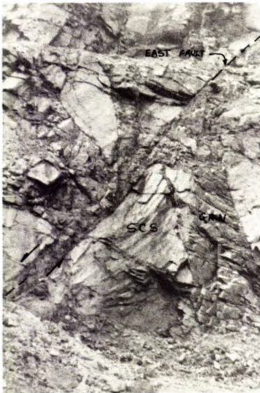
Fig 5 - East fault with a displacement of 20 ft (6 m).
