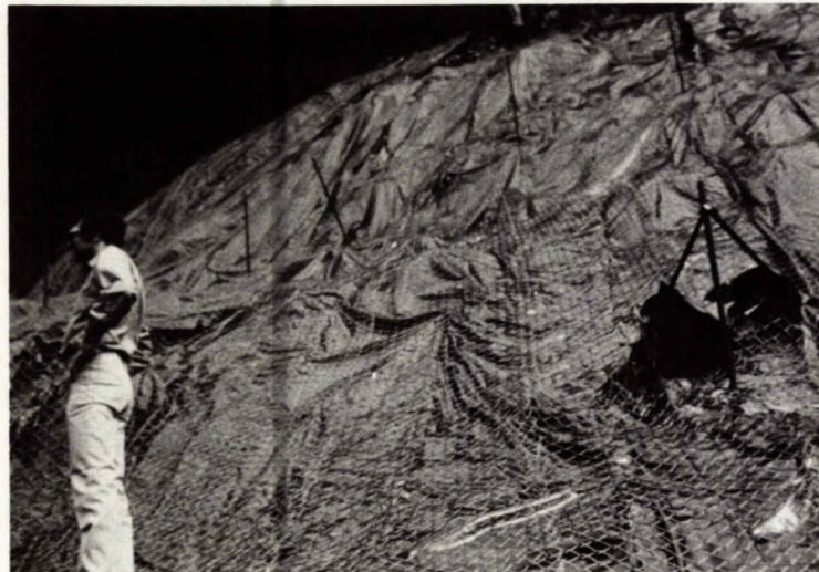
Fig 49 - PVC Sheeting used to prevent water infiltrating a slope.
