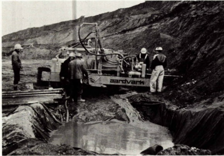
Fig 48 - Track-mounted drilling rig for installing horizontal drains.
