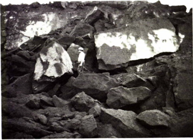
Fig I-3 - Poor blasting fragmentation attributed to permafrost.
