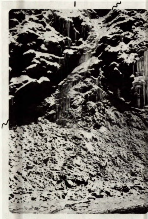
Fig I-12 - Accumulation of ice resulting from seepage of groundwater along the Water Fault at Clinton Mine.
