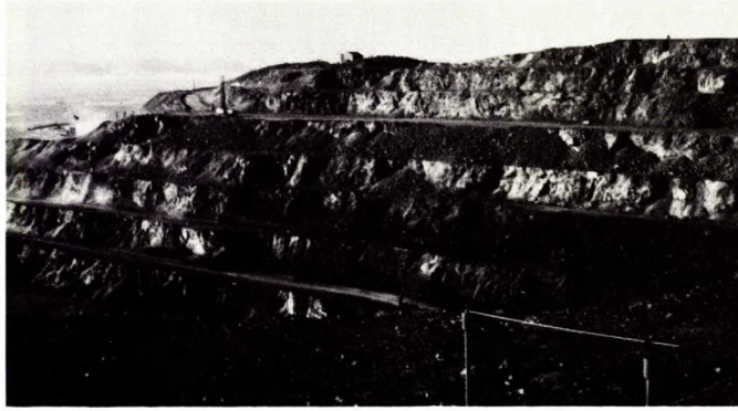
Fig 39 - NorthWall of Iron Monarch Mine with surrounding plain in background. Upper benches are in jaspilite, lower benches are in the amphibolite of the North Wall Dyke Zone. Loose covering 4th face from top is due to cutting-back operations. Crude extensometer in foreground is across a crack formed by minor slide on the south-east wall.
