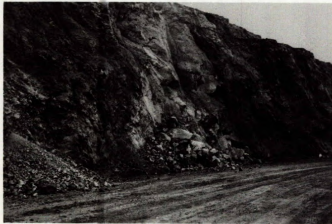
Fig 43 - Face in deeply weathered feldspathic schists on the west wall. Small rock fall developed along shears dipping towards the pit.
