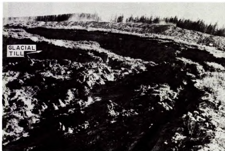
Fig 47 - View looking north of Slide No. 1 from the pit crest at elevation 3725.
