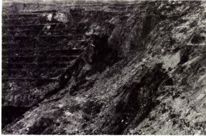
Fig 16 - Rotational shear; within the altered weak rock mass shown in the foreground, instability developed along a circular slip plane.
