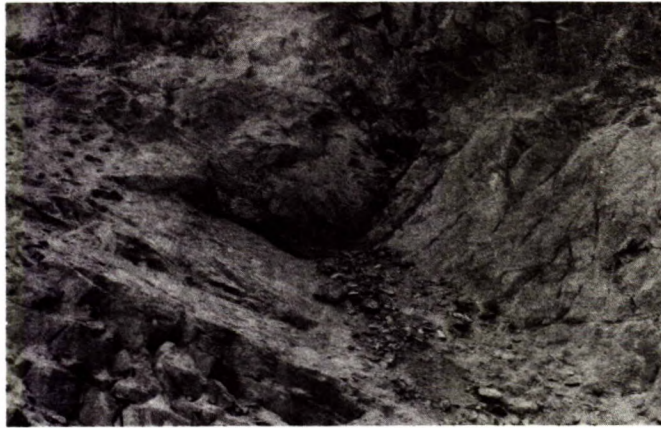
Fig 7 - Wedge sliding; 3-d-wedge instability developed when shear strengths along the weakness planes, oblique to the face, were exceeded.
