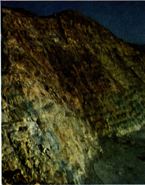
Fig. 9 - A 55° slope 680 ft (207 m) high, which proved to be quite stable.
