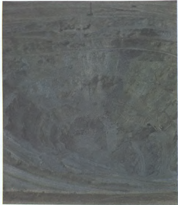
Fig. 31 - A 500 ft (153 m) high slope where the slope angle was limited to 45° because of the development of loose rock on the bench faces.
