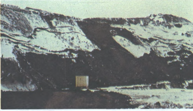
Fig. 29 - A large area involved in a rotational shear slide moving in spite of sub-zero temperatures.
