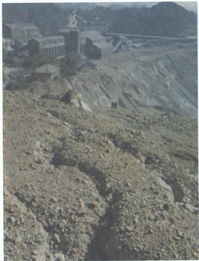
Fig. 48 - A crusher uncomfortably close to the edge of the pit, after many years of expanded mining, where it could be affected by wall instability.
