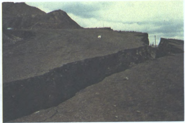
Fig. 47 - A main ramp broken up by wall instability. The haulage system had to be redesigned to route the ore at extra cost up the opposite wall.
