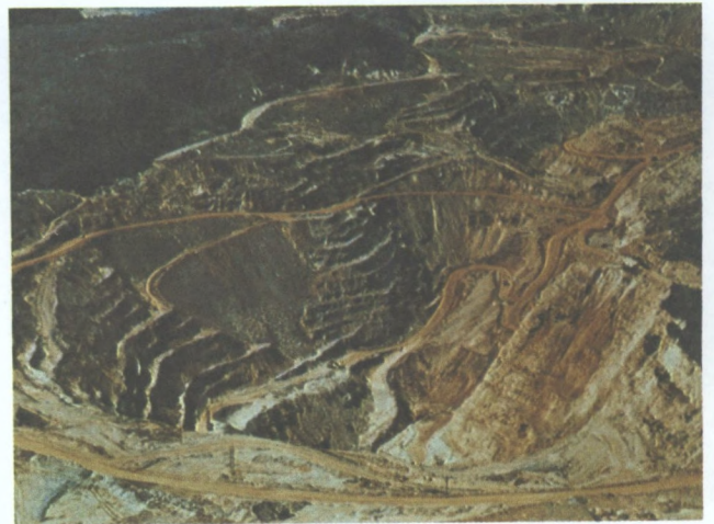
Fig. C-7 - A pit wall that was designed based on analysis of slides in two previous pits in the same formation. The slide that can be seen in the centre of the wall occurred two months after mining was completed and after a scavenging operation had cut the toe back beyond the ultimate wall line.
