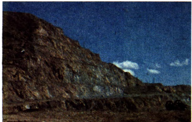
Fig. 6 - A 275-ft (84-m) high 60° slope where it was found difficult to maintain adequate catch benches.
