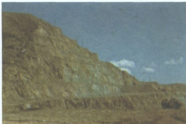
Fig. C-14 - A trial slope to determine if it would be feasible to maintain 60^\circ for a depth of 1000 ft (305 m). It turned out that it was difficult to maintain adequate catch benches.
