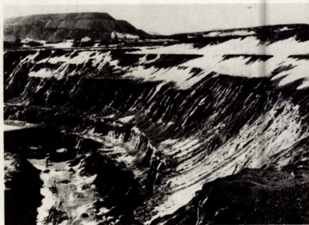
Fig. 1 - Variability in a pit wall. A slide occurred at a section to the right of the photo that was not visually different from adjacent sections. The slide was impossible to predict with certainty, but it had been shown in the design analysis that there was a 10% probability of instability in the entire wall.
