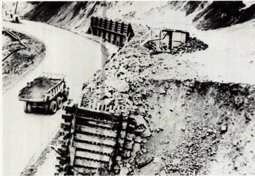
Fig 51 - Longitudinal view of IOC buttress.
