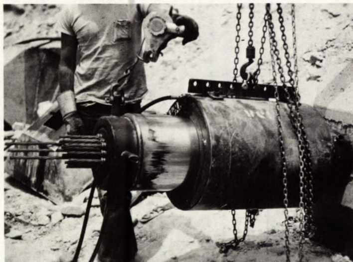
Fig B-15 - A pre-stressing jack tensions a large capacity rock anchor.
