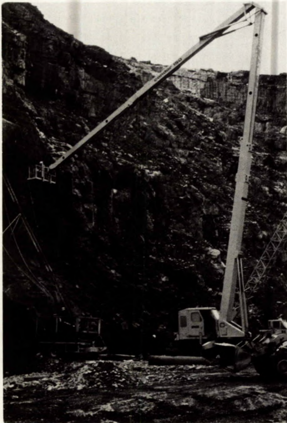
Fig E-2 - The Condor mobile platform used for access to the east wall.
