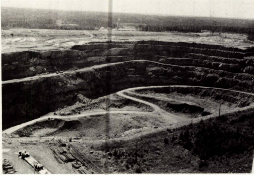
Fig E-1 - General view of east wall of Pipe mine.
