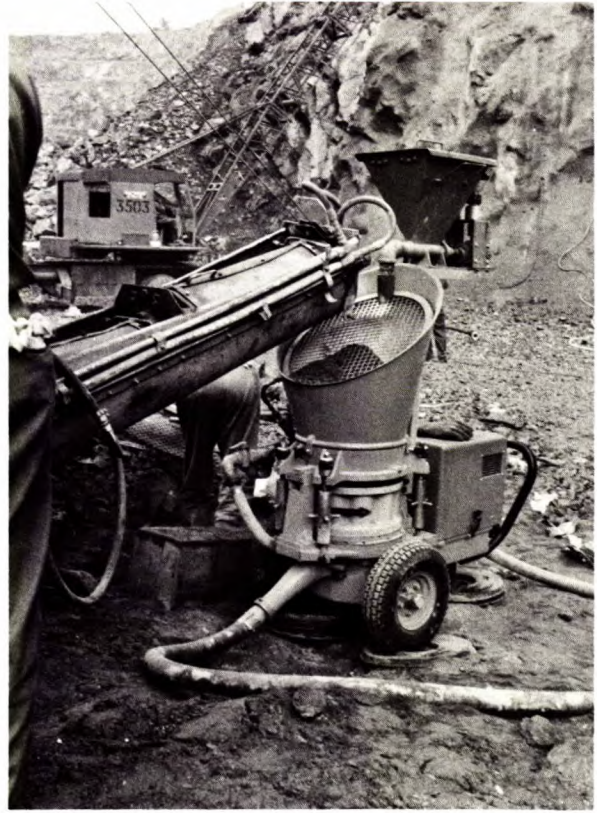
Fig C-4 - The Aliva Shotcrete Machine.
