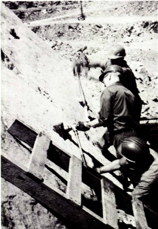
Fig 9 - Torque wrench for tensioning bar rock anchor.
