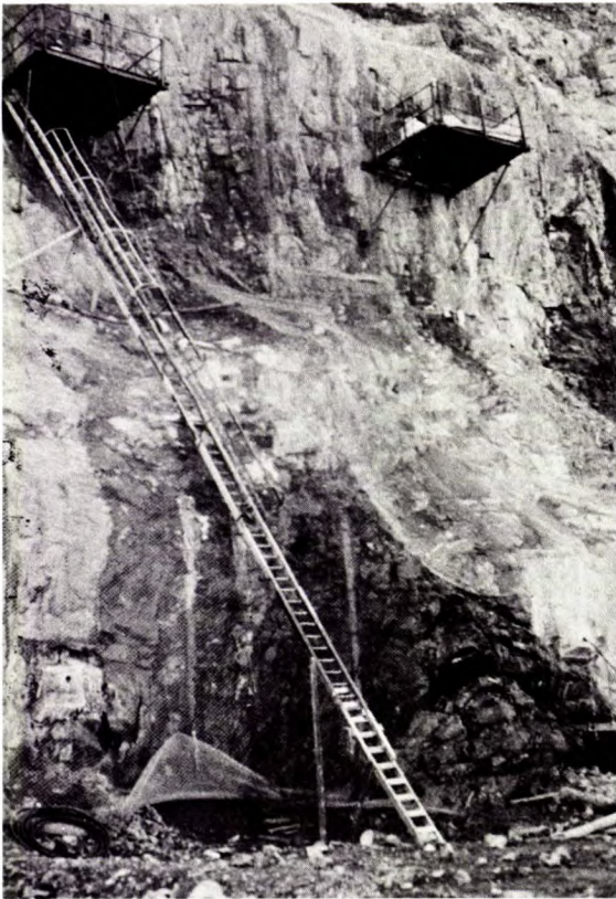
Fig E-8 - Completed platforms for drilling.
