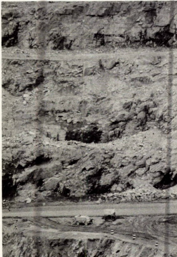
Fig E-6 - Scaling the east wall with a slusher.
