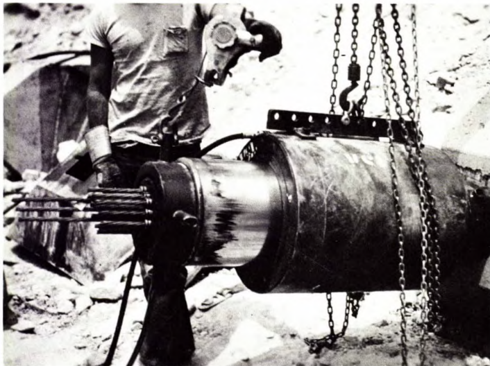
Fig 33 - A large capacity rock anchor being tensioned.
