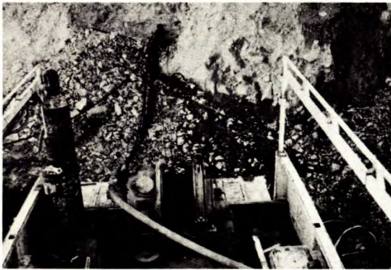
Fig. 23 - A mechanical tugging to aid anchor insertion
