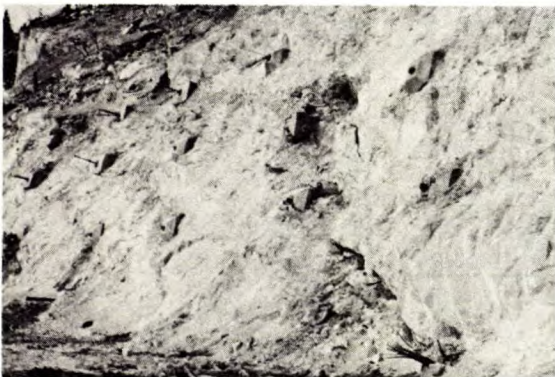
Fig. 31 - Undercut Agua Zarca-Cutler formation showing draining water
