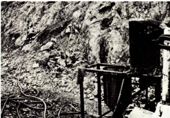
Fig. 24 - Grouting of an anchorage section
