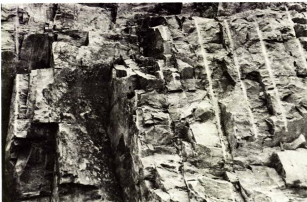
Fig 50 - Open joints at 90° to rock face.
