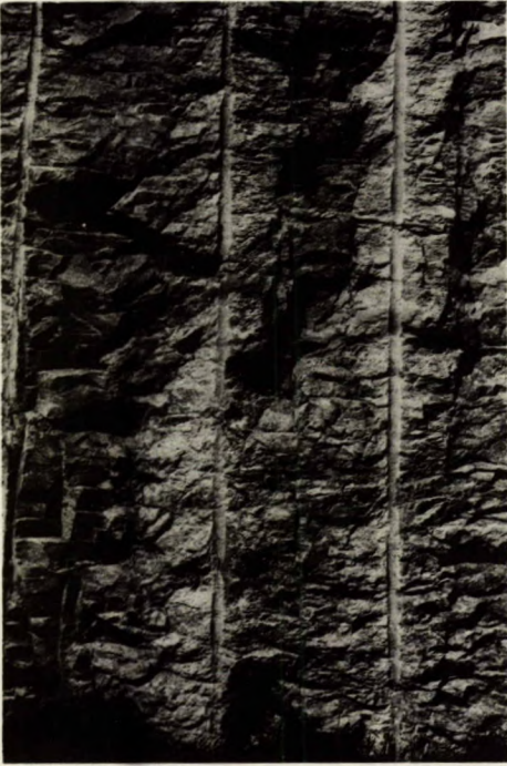
Fig 45 - A good clean pre-split in jointed rock.
