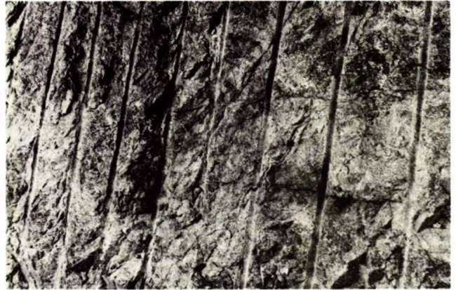
Fig 43 - A smooth clean pre-split surface in competent rock.
