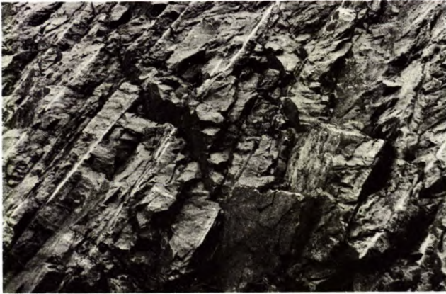
Fig 49 - Steeply dipping joints striking parallel to rock face but not undercut.
