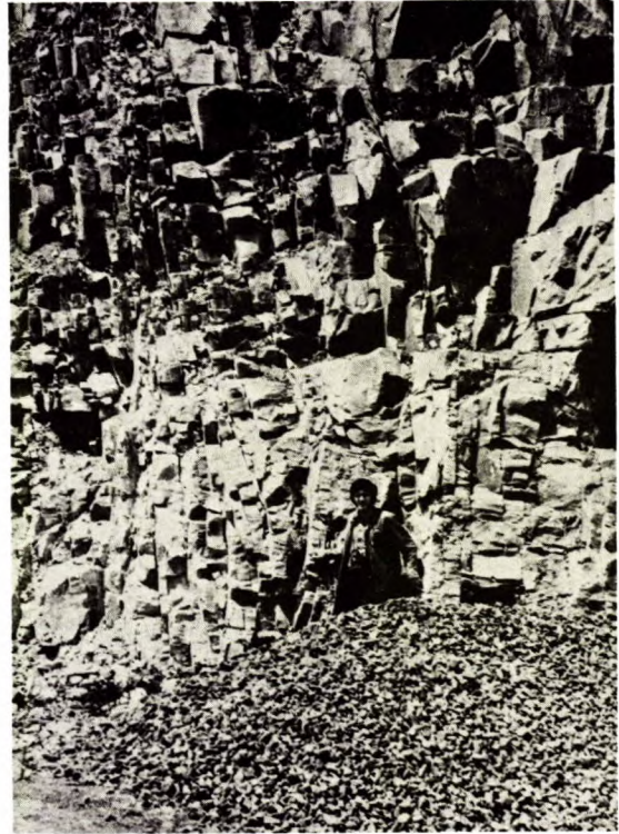
Fig 51 - Frequent vertical jointing at 90° to rock face.
