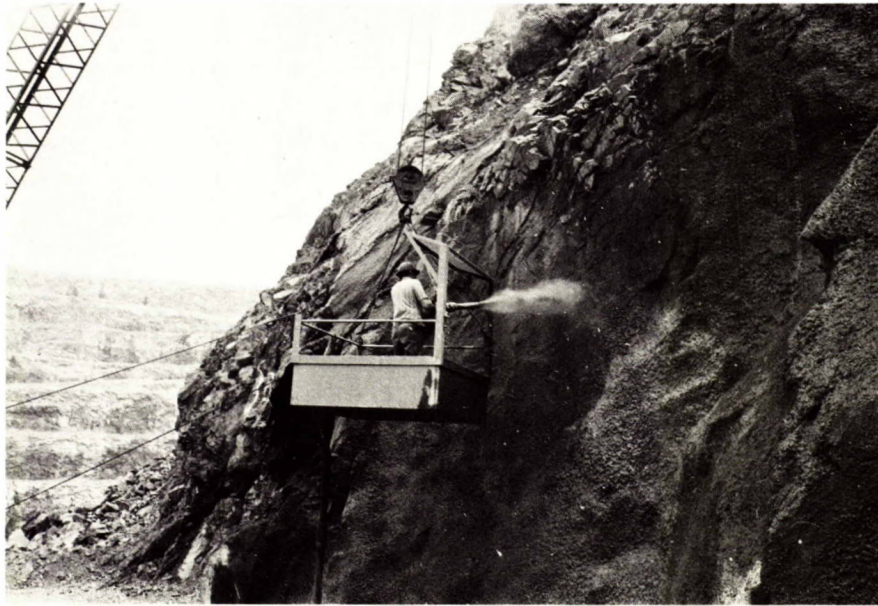
Fig 37 - Applying shotcrete to stabilize a pit wall.
