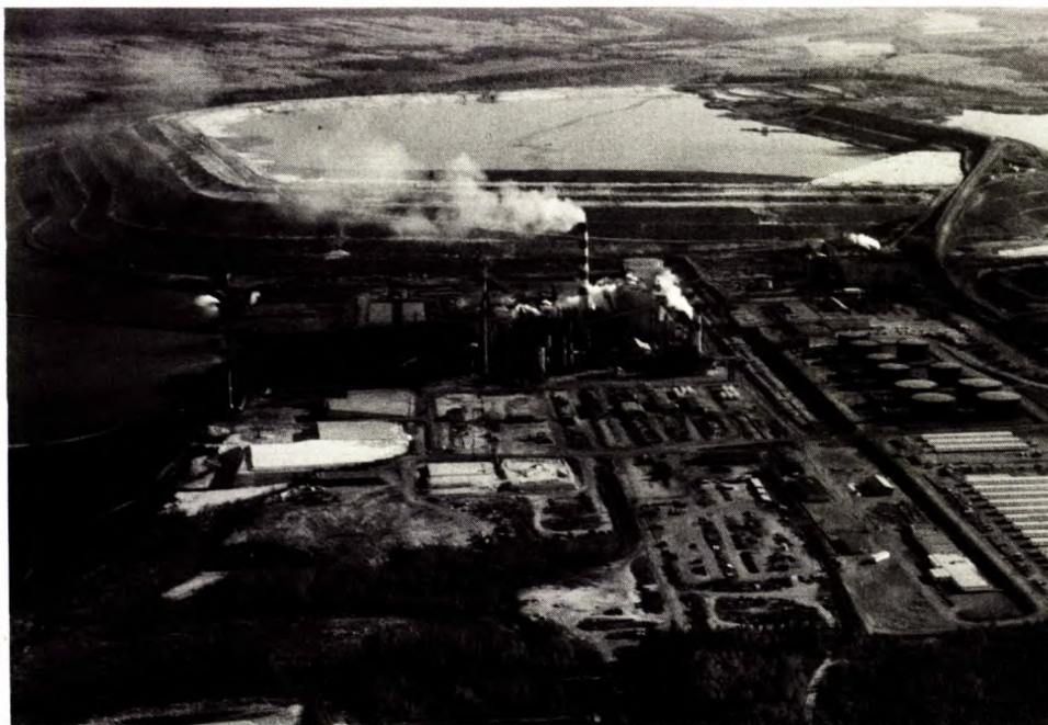
Fig. 16 - The Great Canadian Oil Sands Limited facility near Fort McMurray, Alberta -- an example of a pioneer commercial plant. Operating experience in this plant, the first commercial-scale oil sands installation in the world, has helped engineer larger plants such as Syncrude (Fig. 17).
