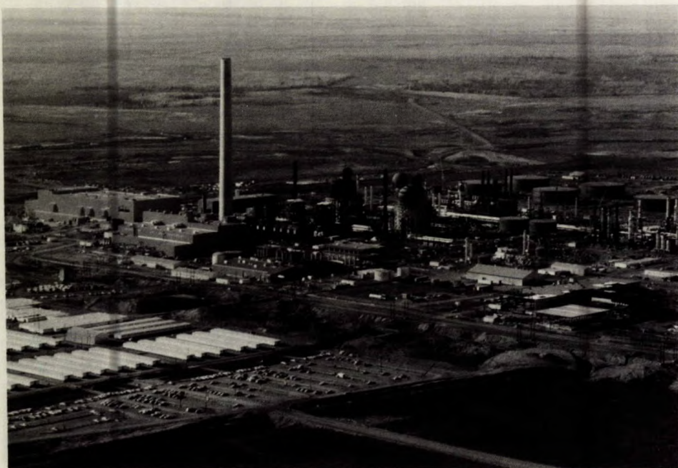
Fig. 17 - The Syncrude Canada Limited oil sands plant during construction near Fort McMurray, Alberta, a full-scale commercial installation. In developing technology from the bench scale (Fig. 15) to this scale, several intermediate steps may be involved: small pilot, large pilot, demonstration, and pioneer commercial (Fig. 16). Decisions on when or whether to proceed to the next stage are crucial as large investments in time and money are involved.
