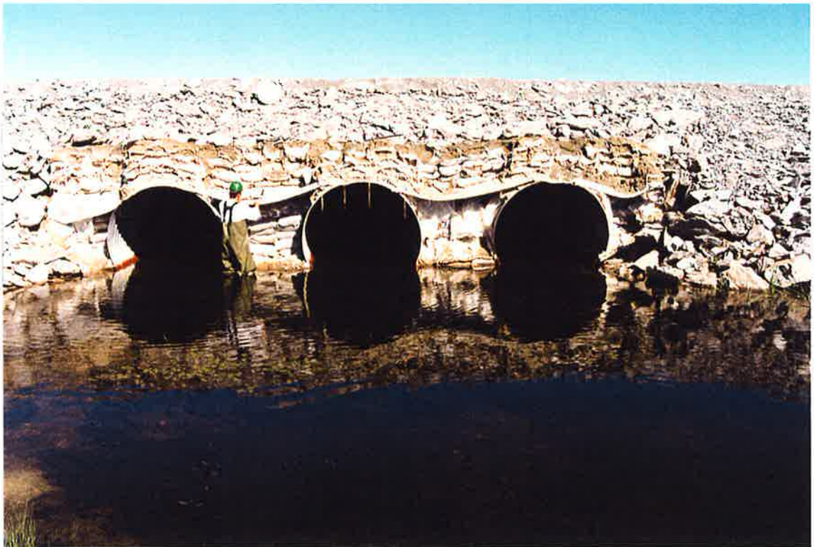
Photo 8. Flow measured at road culverts at lower end of exposure area
