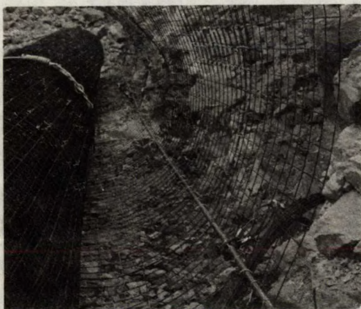
23. Wire Roll Anchored Temporarily by Short Bolts.
