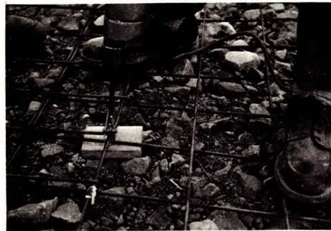
20. Wire-Twisting Device in Use.
