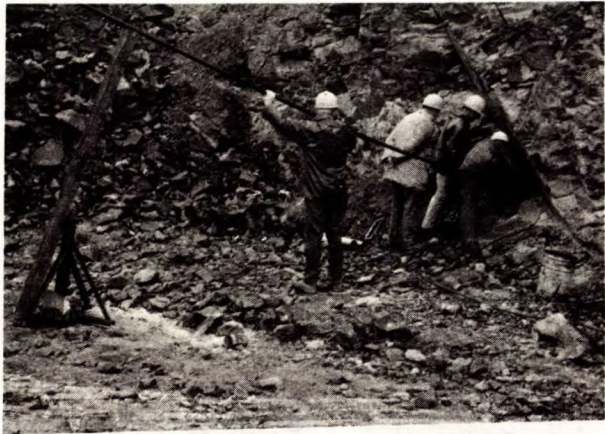
17. Installing the Stressteel Rod.
