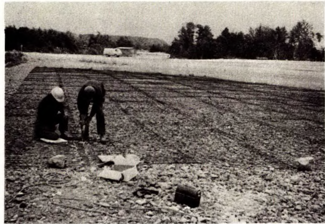
18. Mesh Lengths Laid Out and Wired Together on the Surface.
