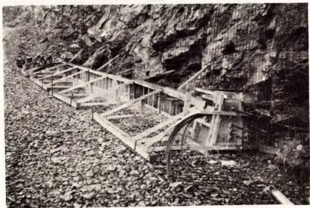
27. Form Work for Horizontal Concrete Stringer - Lower Bench.
