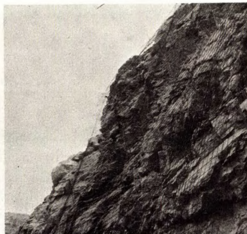
26. Wire Mesh in Position.
