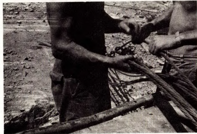
12. Cable Anchor Assembly- Positioning the Strands on the Spacer.
