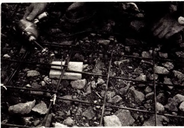
19. Wiring Mesh Sections Together (Showing Wire-Twisting Device).
