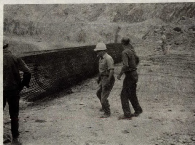
24. Wire Mesh Rolled Over Bench Edge.
