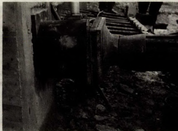
38. Load Cell Between Concrete Pad and Tensioning Jack,
