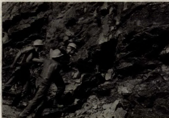
14. Installing the Cable.
