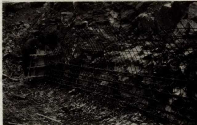
30. Form Work for Anchor Pads on Top Bench and Steel Bar Horizontal Stringer,
