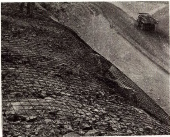
25. Wire Mesh in Position.
