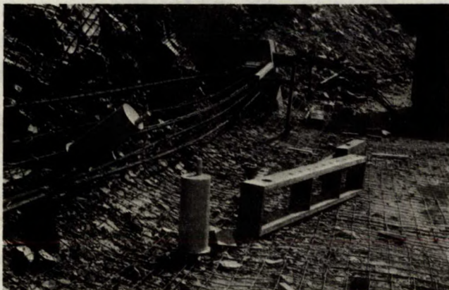
31. Extensometer Installations (Top Bench).
