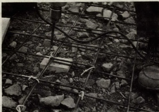
21. Wire-Twisting Device in Use.
