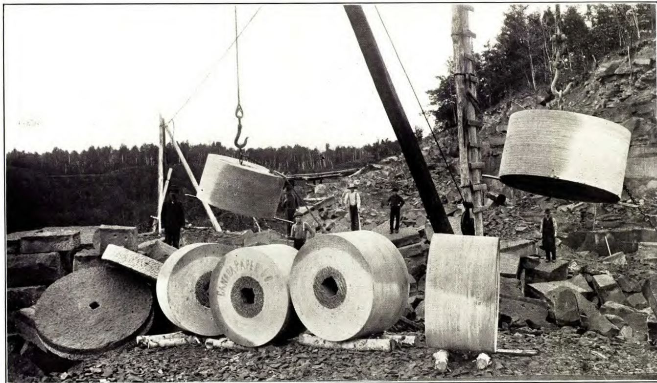
French Fort quarry, Newcastle, N.B., (1897). Finished pulpstones and semi-finished grindstones.
