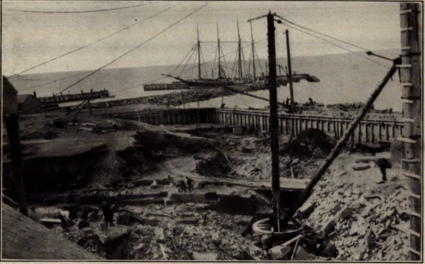
A. Read Stone Company's grindstone quarry, Stonehaven, N.B. General view of quarry and dam, looking northwest.
