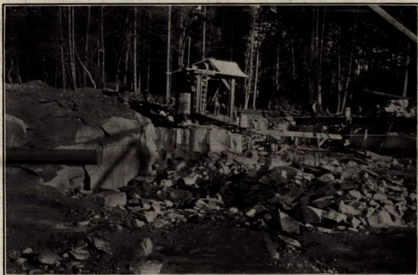
A. The McDonald pulpstone quarry, Newcastle island, B.C., showing cylindrical cutter and driving gear.
