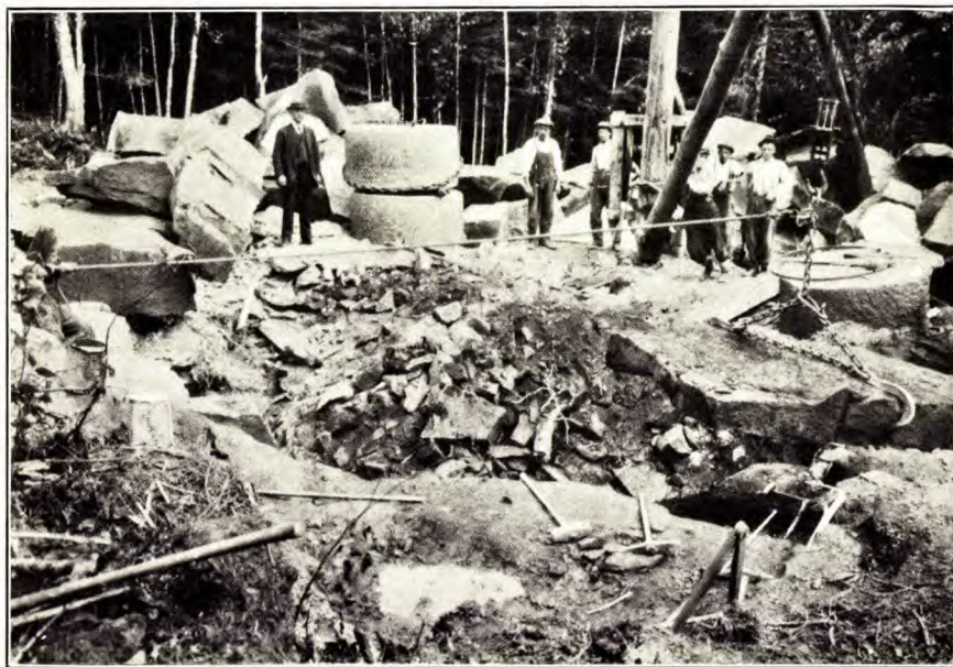
B. Read Stone Company (Dobson quarry), Rockland, N.B. Lifting out a grindstone slab.
