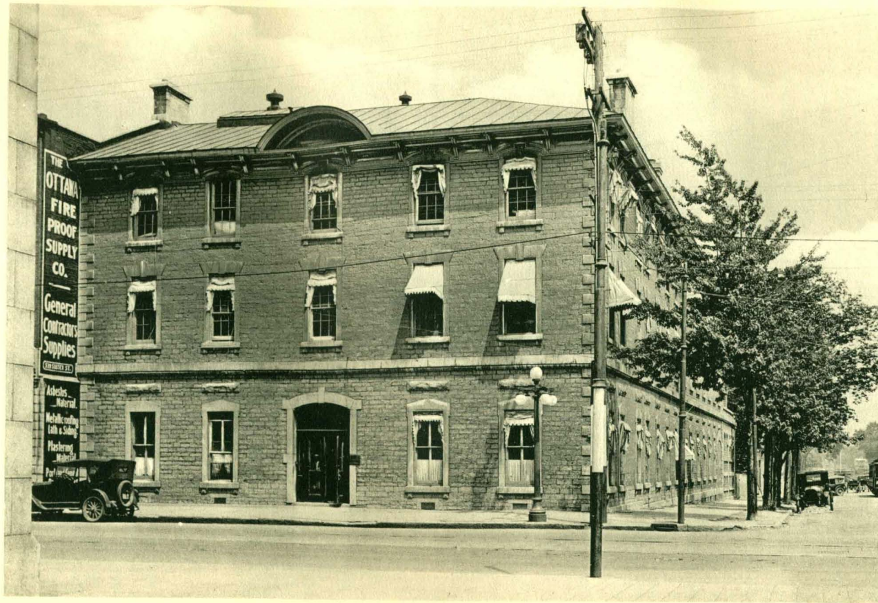
Former Geological Survey office and Museum on Sussex street, Ottawa, to which the Geological Survey moved from Montreal in 1880. Now occupied by the Mines Branch.
