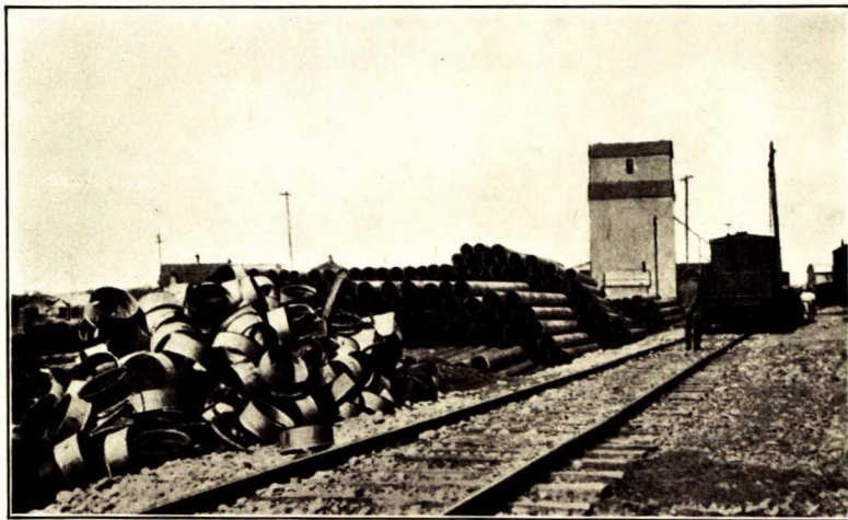
Scene at Okotoks, Alberta, showing pipe for main line of Coronation Western Natural Gas, Light, Heat, and Power Co., Ltd.
