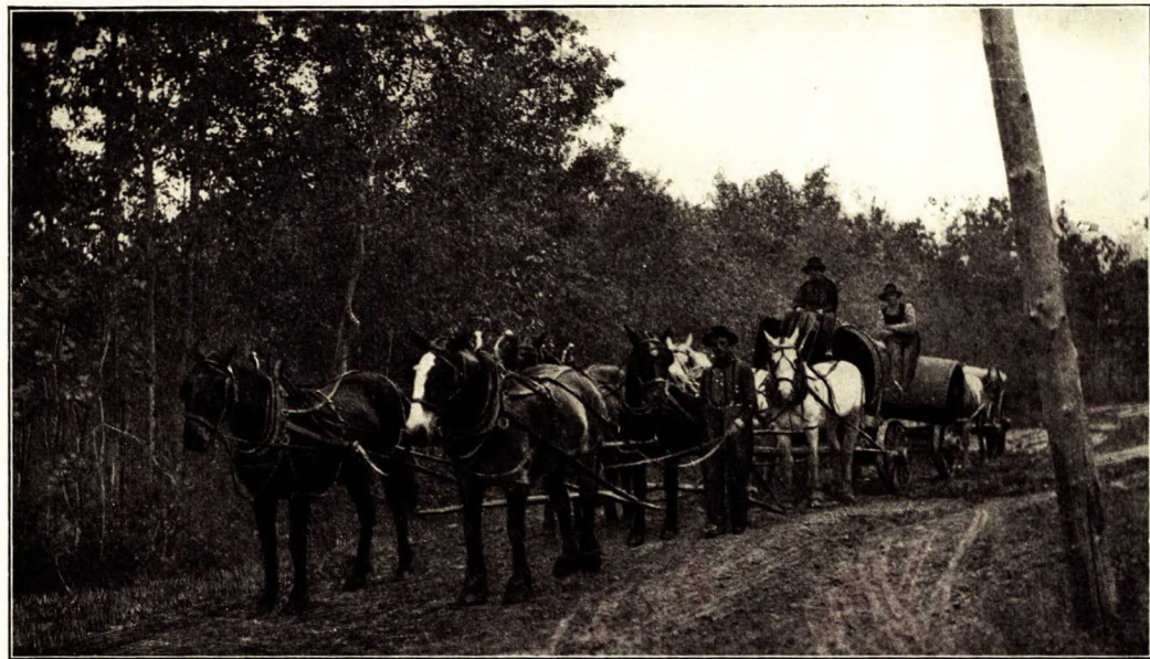
Hauling boiler from Edmonton to Athabaska, Alberta, 1911.
