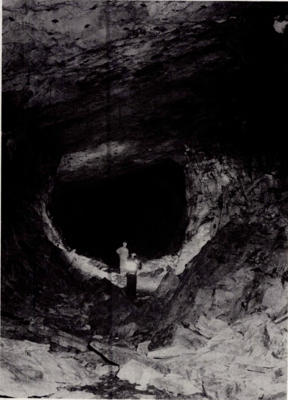
Failing pillars in a rockburst zone at Denison Mine.
