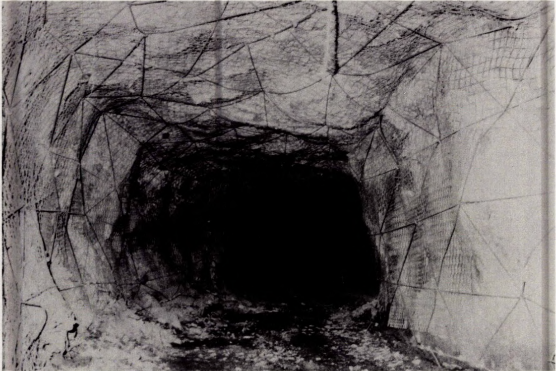
Lacing used in rockburst-prone areas at Strathcona Mine.
