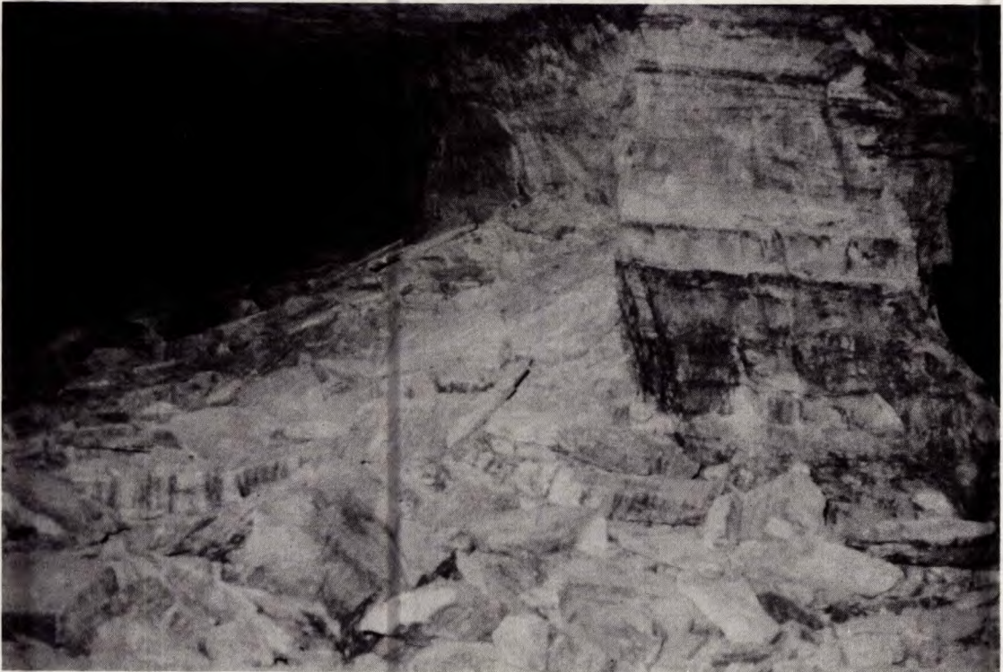
Partial pillar failure at Denison Mine.
