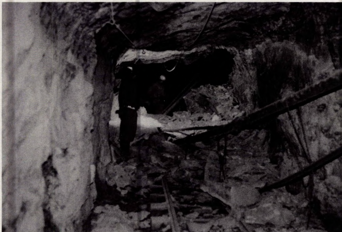
Strain burst in a drift at Quirke Mine.
