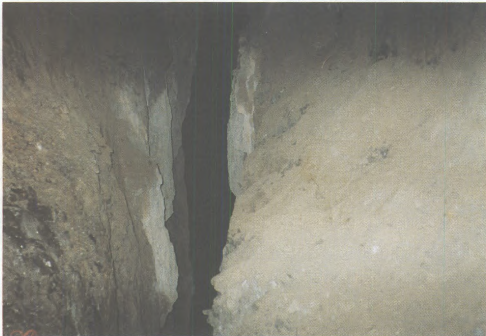
Crown pillar at the Campbell Red Lake Mine, which was destressed then mined using longhole methods.
