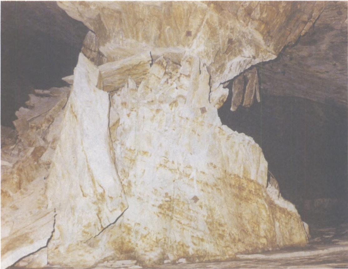
Backfill being poured around a failed pillar at the Denison Mine.
