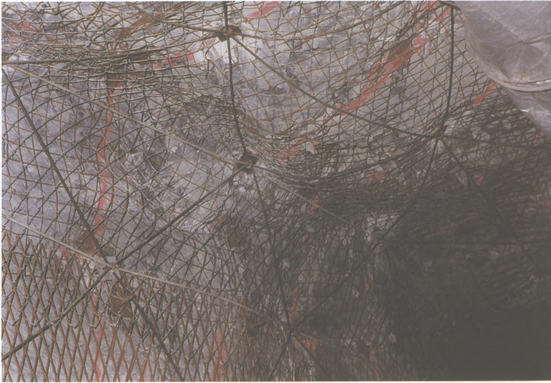
Lacing installed at the Strathcona Mine.
