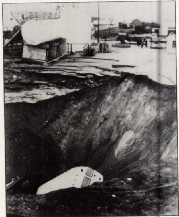
Figure 1 : 1963 Subsidence of some old mine workings beneath a parking area in Timmins, Ontario.
