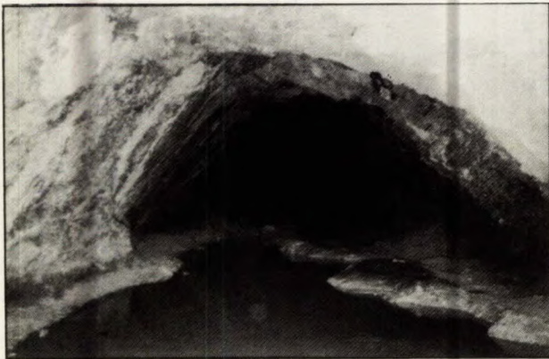
Figure 3 Gallery working in Upper Wenlock Limestone
