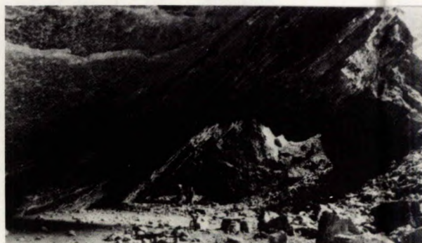
Figure 18 Shallow vaulted roof in Nodular Beds above Lower Wenlock Limestone mine dipping at about 45°
