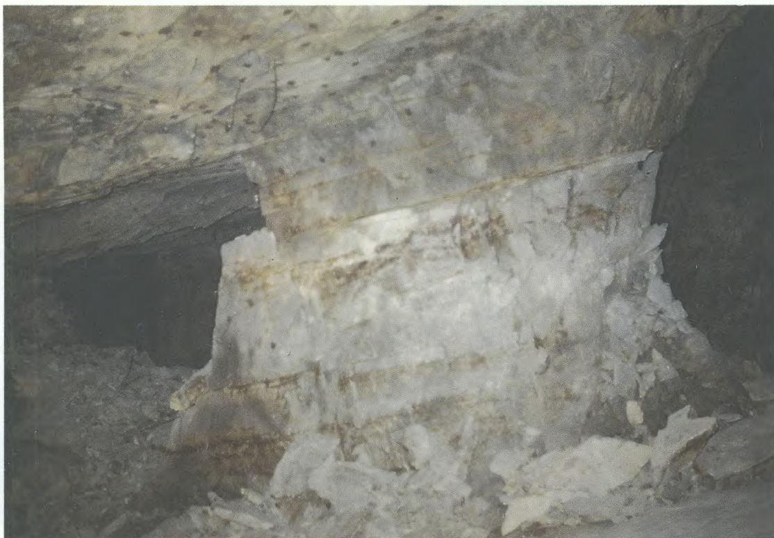
Panel pillar at Denison Mine. The hanging wall appears to have moved up-dip relative to the footwall.
