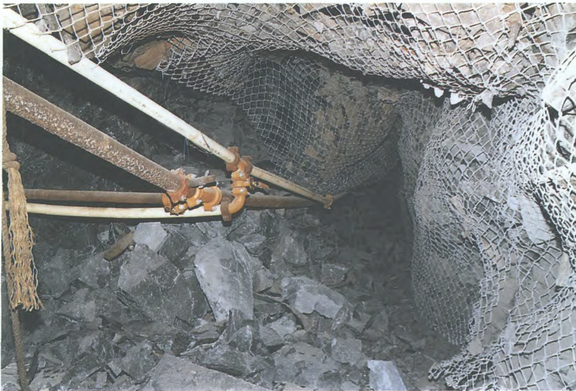
Effects of a 2.5-magnitude rockburst in a waste pillar on the 5600 level at Macassa Mine. More than 400 t of rock were displaced and the drift closed over a distance of 15 m. Note: linked-wire mesh and 2.4-m mechanical bolts held.
