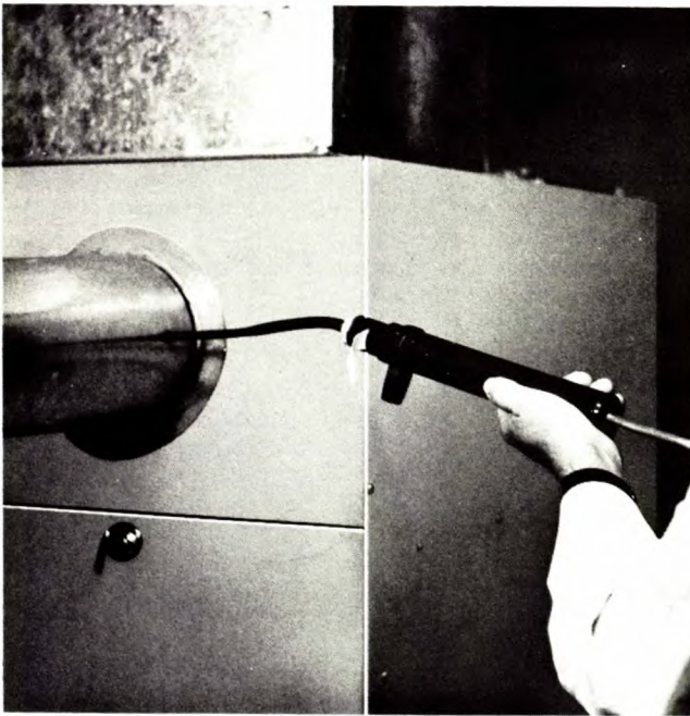
Figure 3.15 Using a smoke tester in a flue pipe
