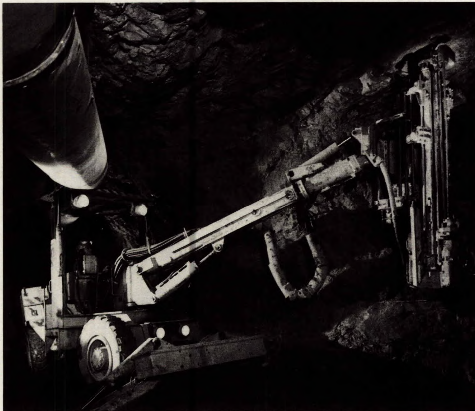
Fig. 72—Automated roofbolter with operator at a safe distance from operation. The boom can extend 1.7 m on this unit
