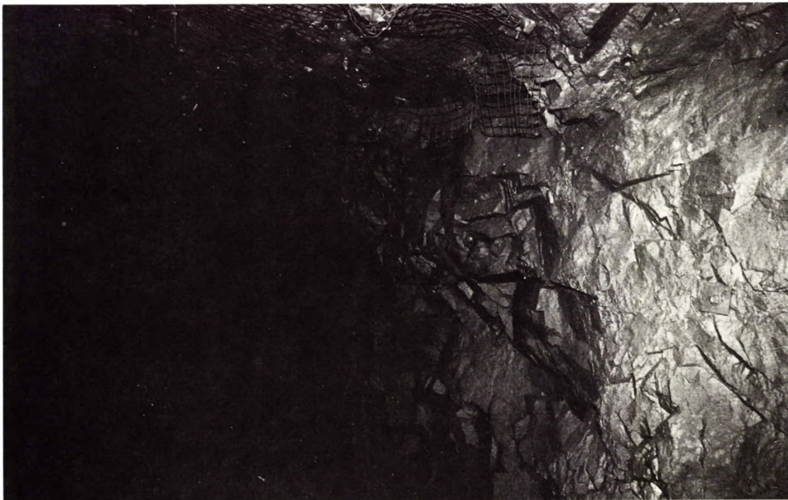
Mine 2, gallery 4: 2.0 fractures/metre, RQD = 98% 3 minor sets, dip = 80°, dip = 45°, dip = 20°
