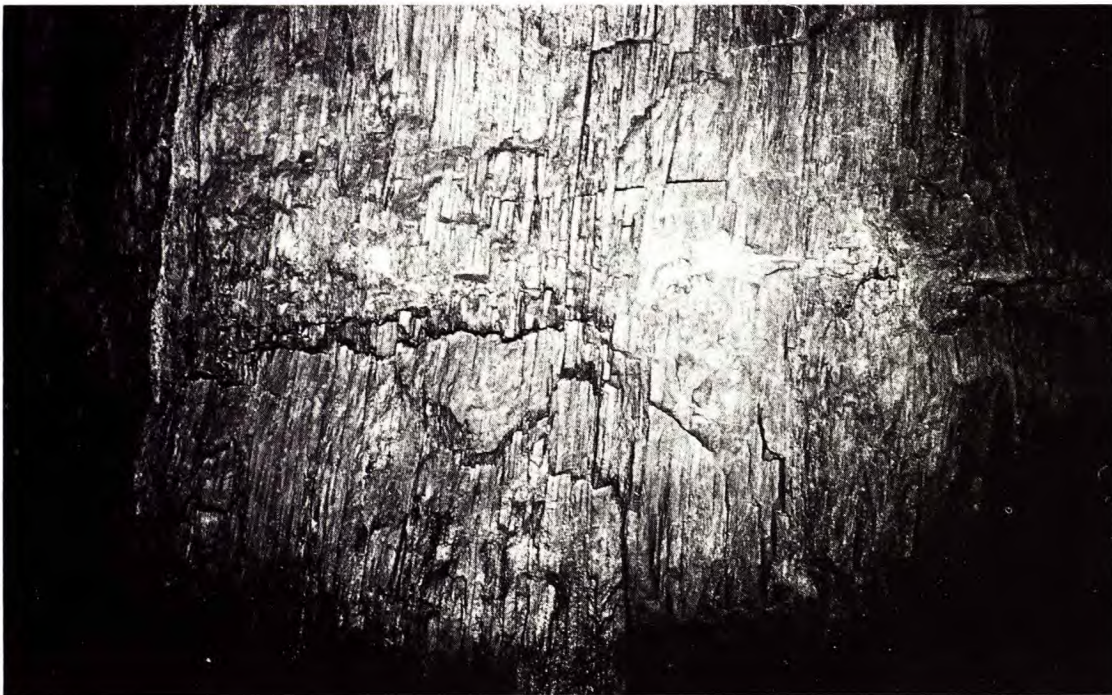
Mine 9, gallery 4: 20 fractures/metre (in this location), RQD = 40% 2 major sets, dip = 90^\circ (schistosity), and dip = 0^\circ
