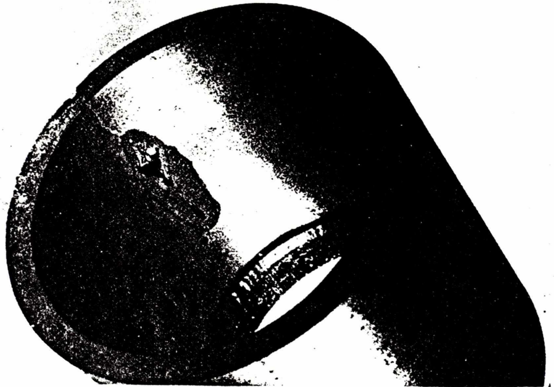
Fig. 3.II Cast iron pipe showing penetration by bacterial corrosion (Crown Copyright reserved)
