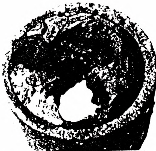
Fig. 3.17. Advanced stage of tuberculation in a section of cast iron pipe
