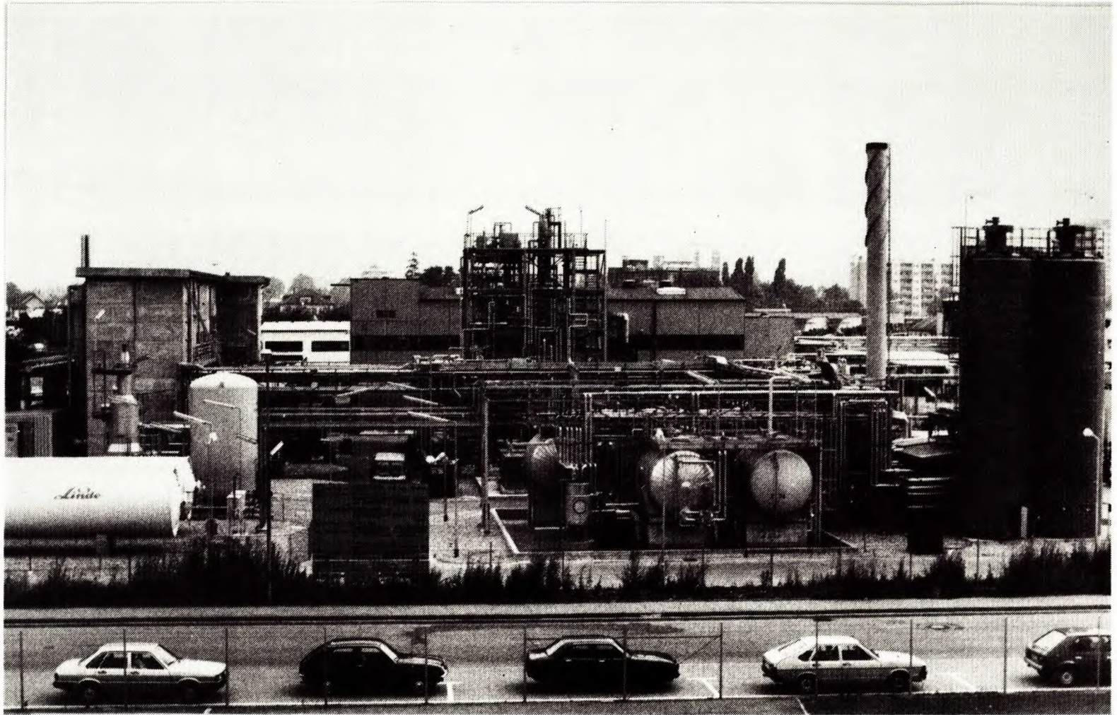
Photo 5 – The 3 t/d pilot plant for coal hydrogenation of Lahr (tubular reactor concept) Source: Salzgitter AG/Imhausen Chemie GmbH
