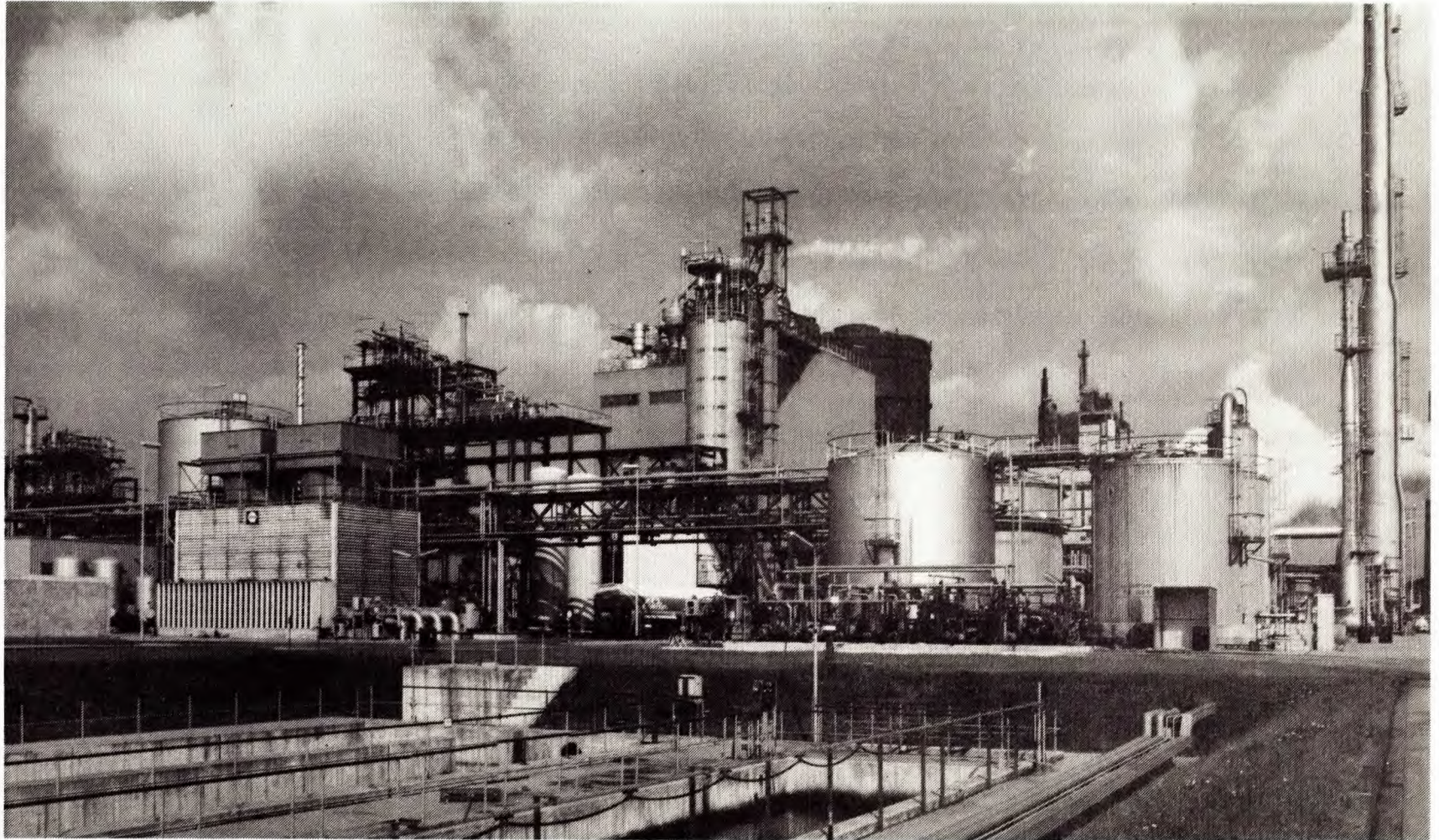
Photo 3 – The 200 t/d pilot plant for coal hydrogenation at Bottrop Source: Ruhrkohle AG/VEBA OEL AG
