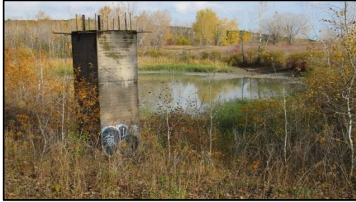
Tailings decant pond
