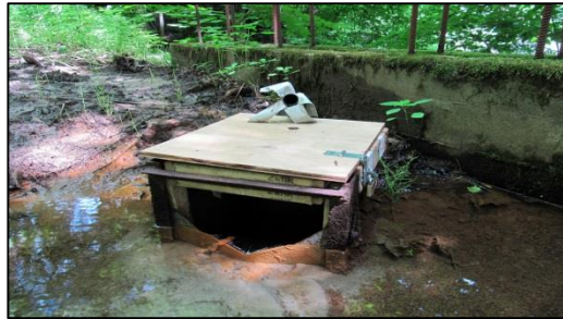
Weir at tailings seepage point
