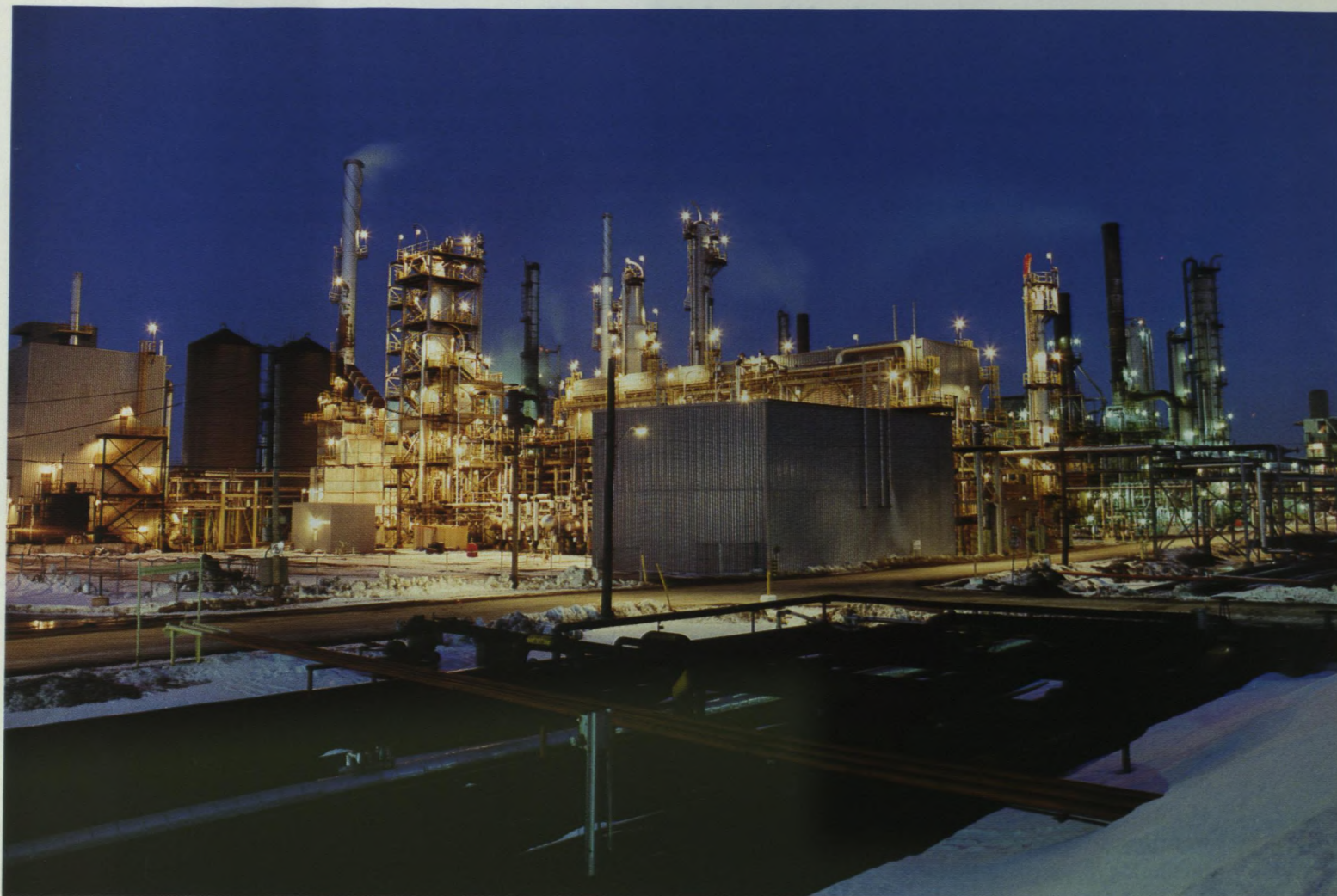
The 5000 b/d CANMET Hydrocracking demonstration plant in Petro-Canada's Montreal refinery uses new generation hydrogen addition technology to convert pitch to distillates.
