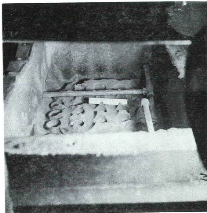
FIGURE 1b Main air heater tube sheet second pass up to 2 - 3 inches of powder.
