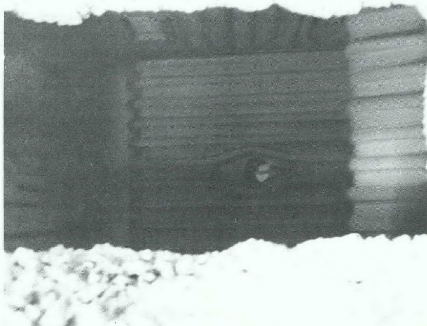
Fig. 8 - Deposits on refractory and water-walls of furnace
