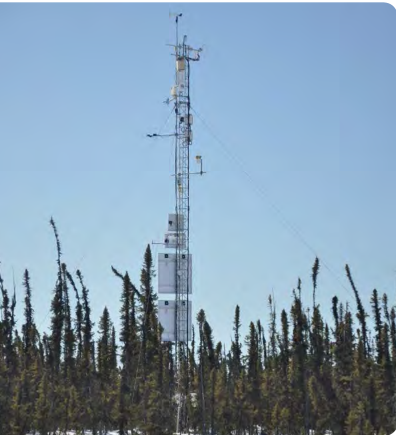
Solar-powered instruments on the tower at Scotty Creek, Northwest Territories, collect data on greenhouse gas and energy fluxes.
