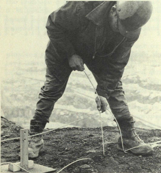
Figure 22. Connecting Primacord downline to a trunk line. (Courtesy Canadian Industries Limited)
