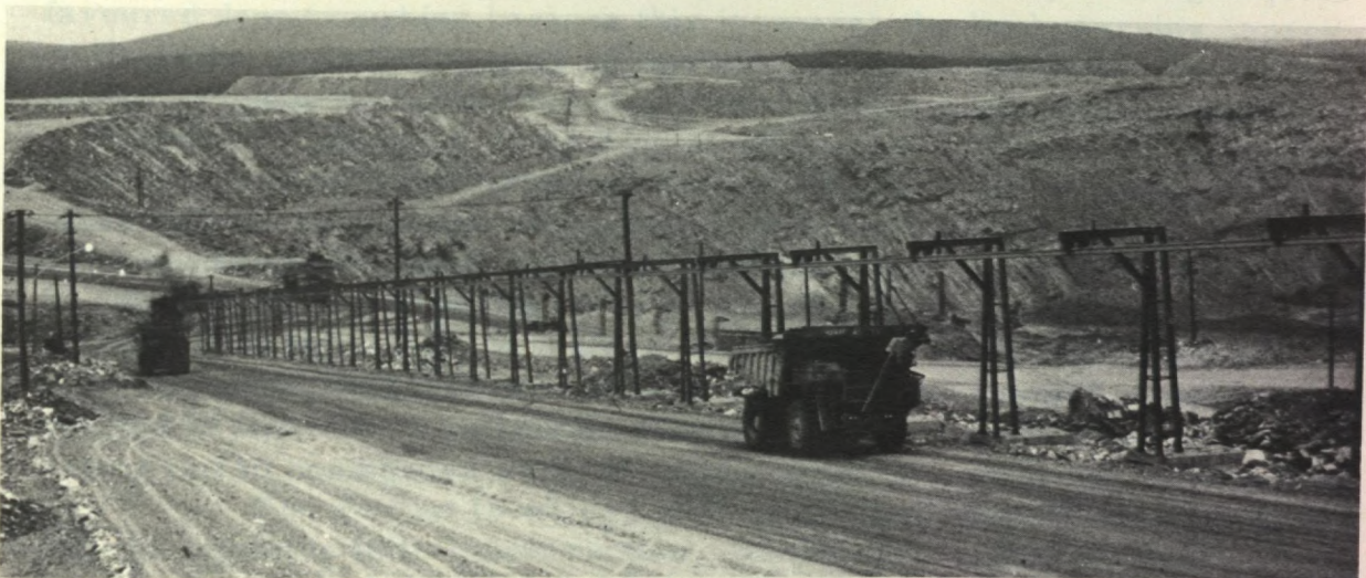
Figure 31. Trolley-assisted haulage on a 10-per-cent grade. (Courtesy Quebec Cartier Mining Company)
