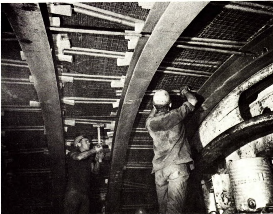
Figure 41. Blocking steel lagging to ringbeams with wooden wedges.
