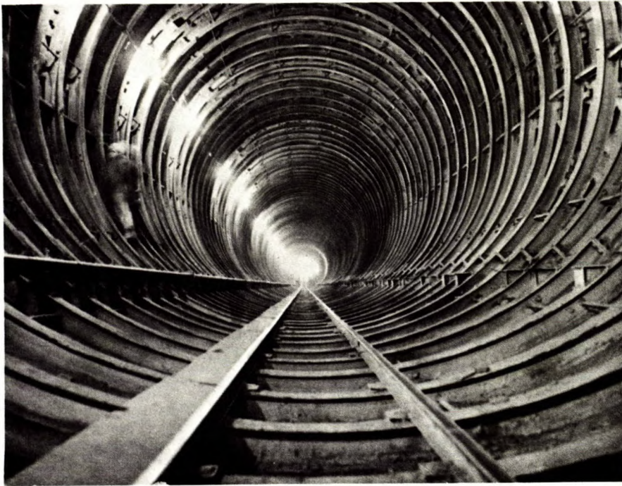
Figure 17. Tunnel section after installation of a temporary ground support system.
