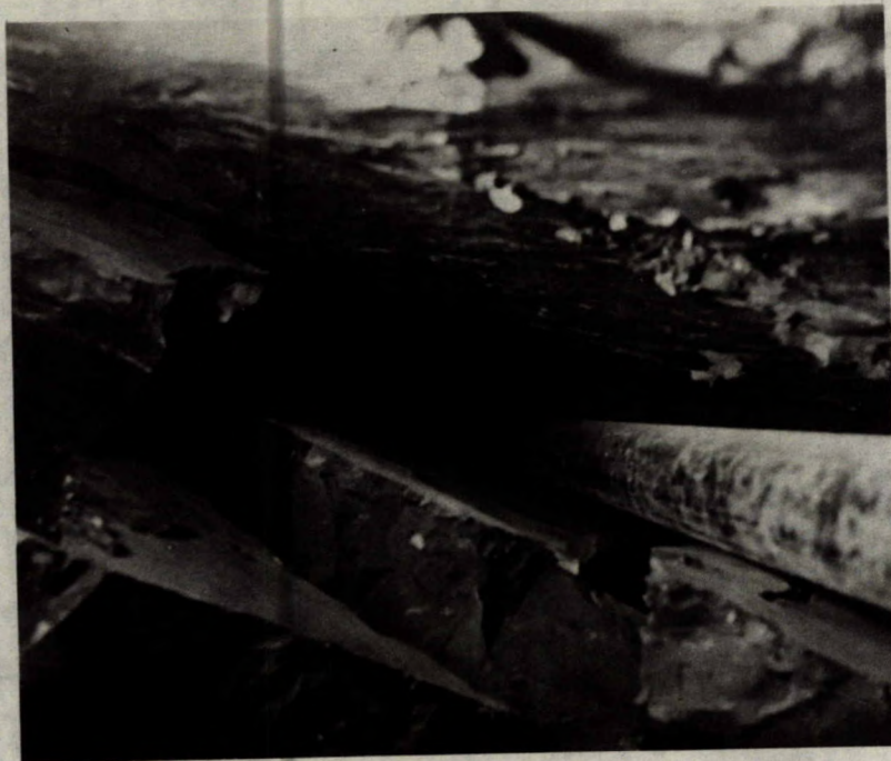
Figure 30. A fallout area with a grout pipe installed.
