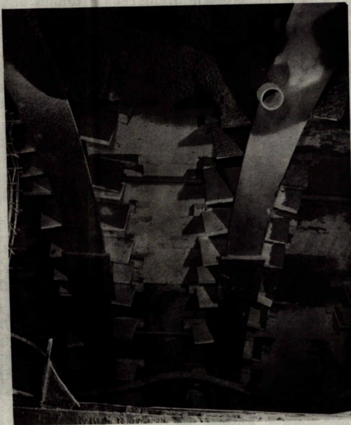
Figure 30. A fallout area with a grout pipe installed.
