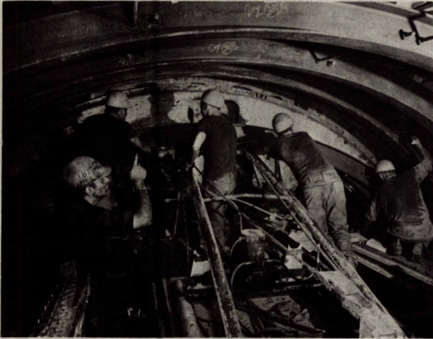
Figure 38. The hydraulically operated ringbeam positioner in action.
