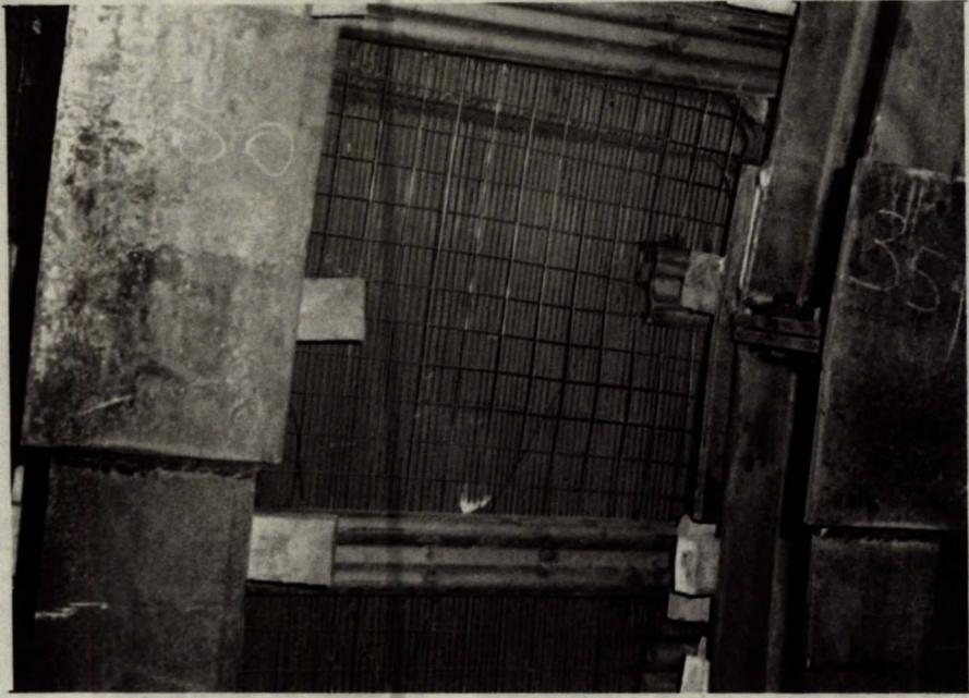
Figure 42. A view of the shale surface before guniting.
