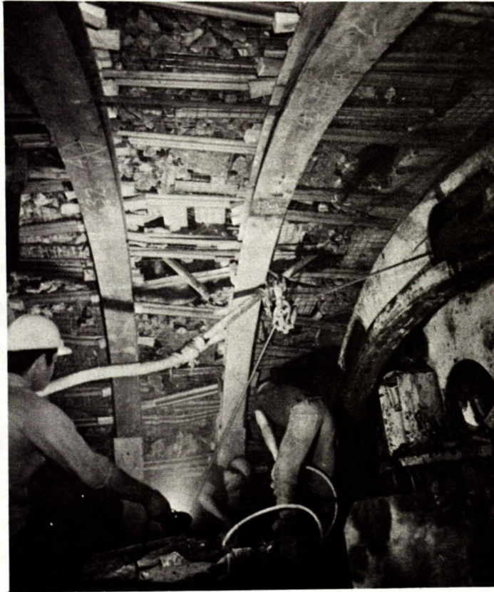
Figure 32. Pumping grout into a fallout area.
