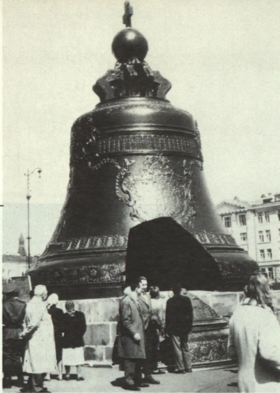
Figure 18. "Tsar-bell" in Moscow, a 220-ton bronze casting (AD 1733)
