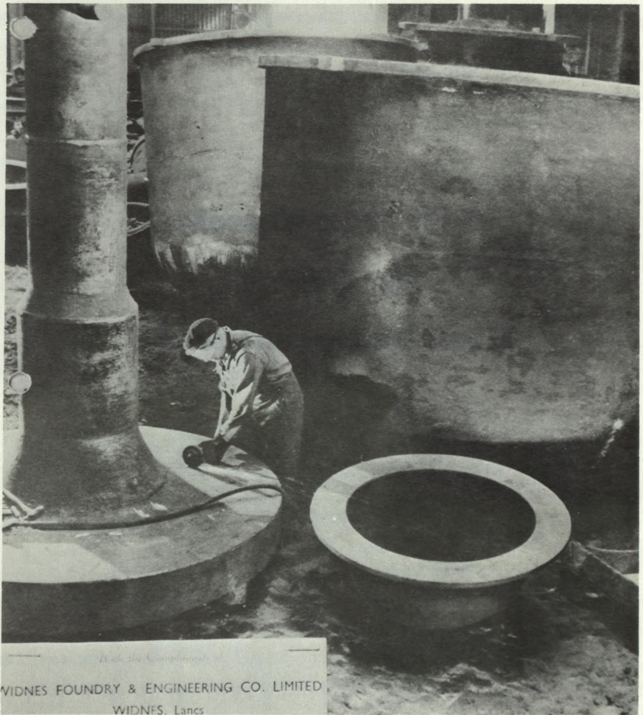
FIGURE 10: LARGE AND SMALL CHEMICAL PROCESSING VESSELS AT MODERN FOUNDRY, 1962
