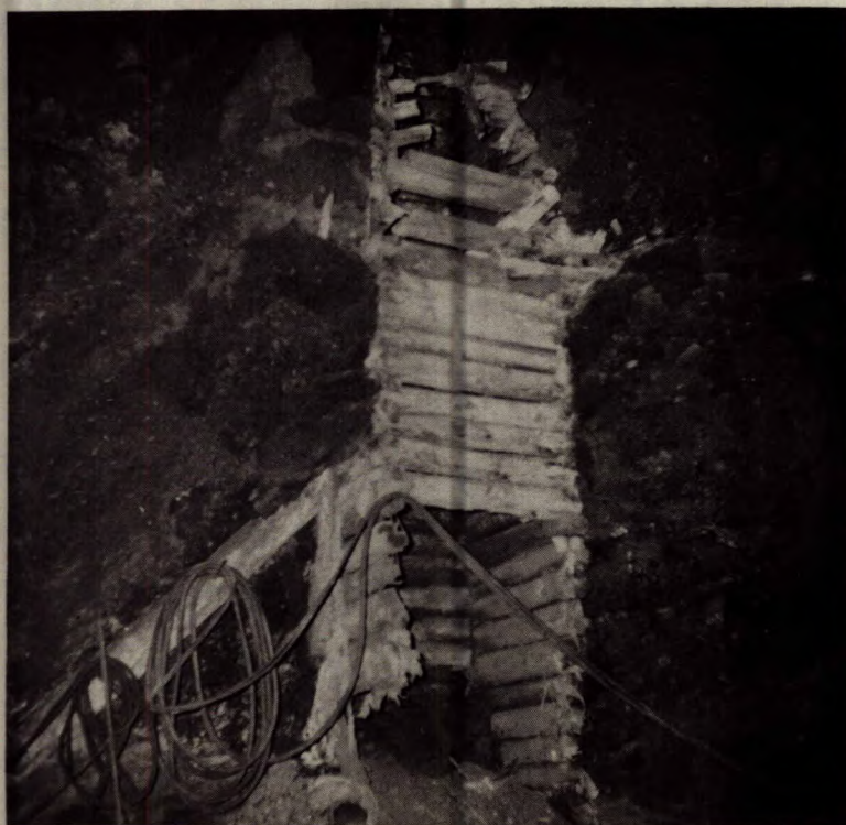
Figure 15. Manway left in consolidated fill.
