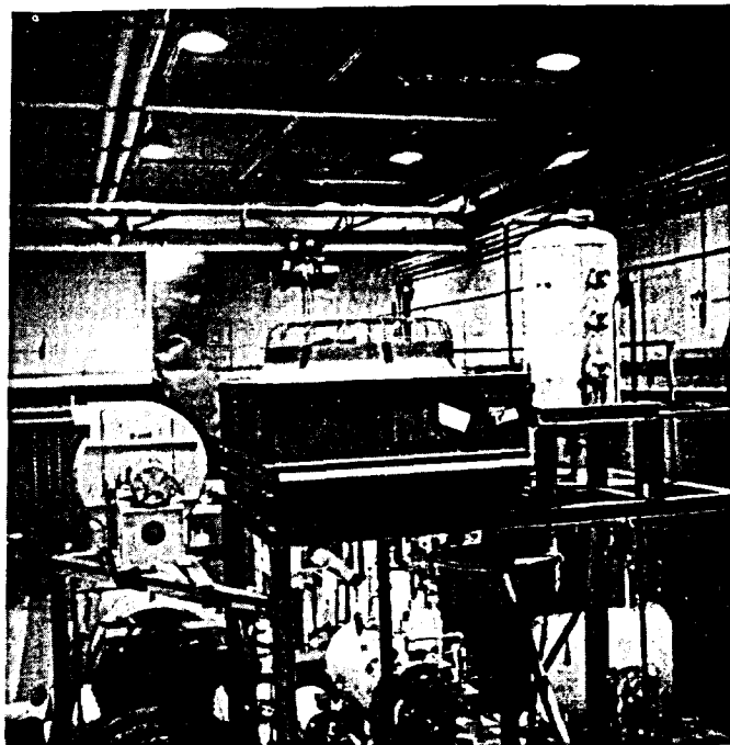
FIG. 8. Flue gas recirculation blower, air-cooled heat exchanger, and expansion tank for the CCRL tunnel furnace.
